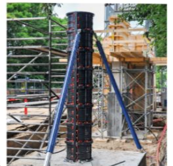
Geotub construction site for railway footbridge Aarsland, Denmark
