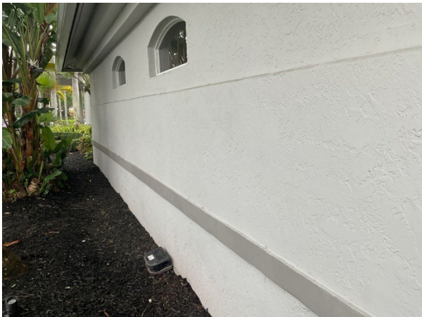
Stucco wall finishes
