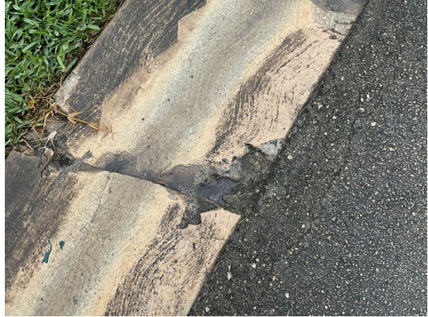
Concrete spalls
