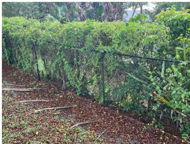
Chain link fence
