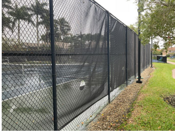
Chain link fence
