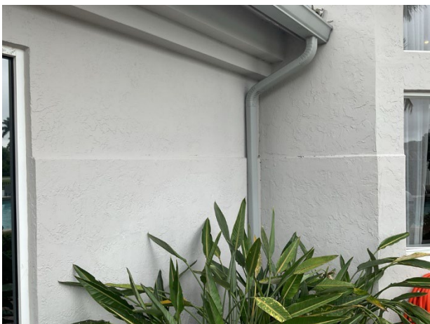
Stucco wall finishes
