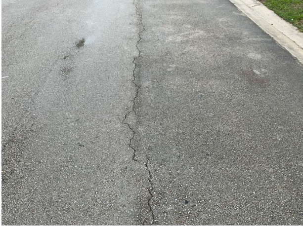
Pavement cracks
