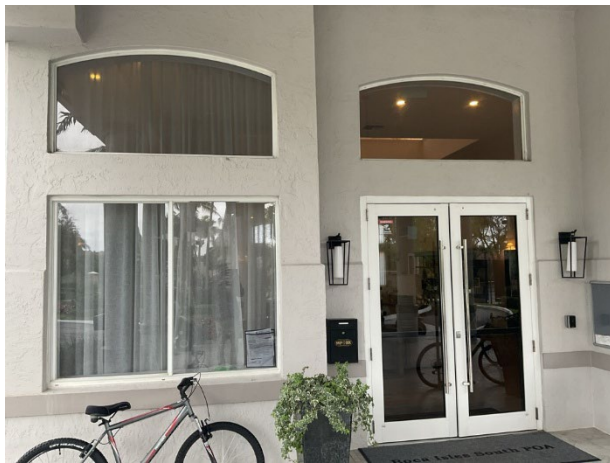
Common windows and doors
