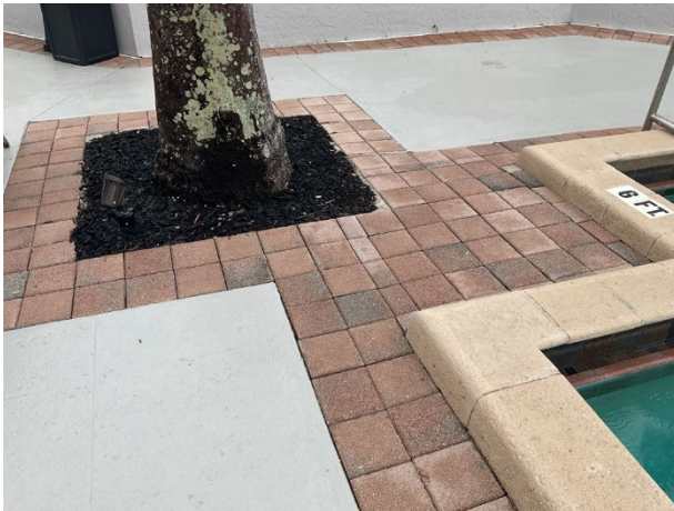
Paver pool deck overview
