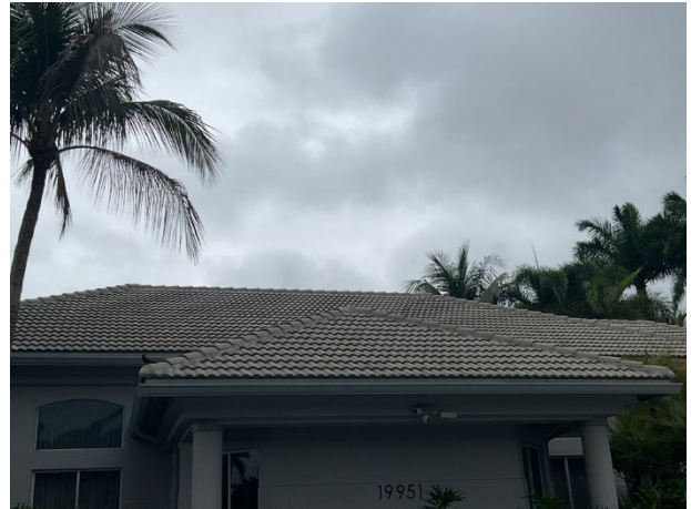
Concrete tile roof at clubhouse
