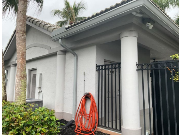
Aluminum gutters and downspouts
