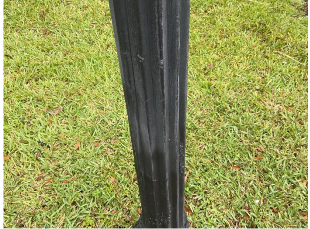
Finish deterioration
