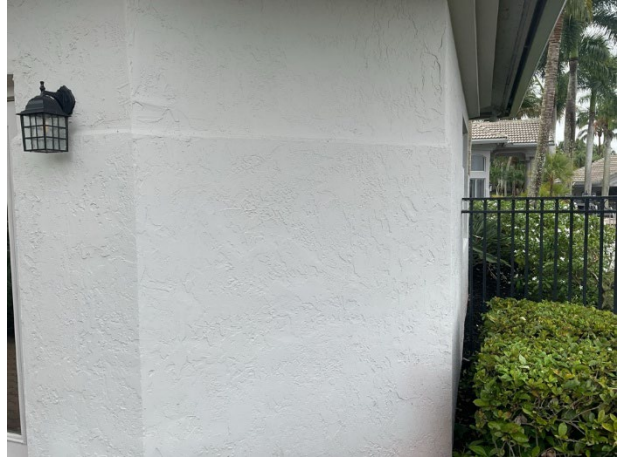
Stucco wall finishes
