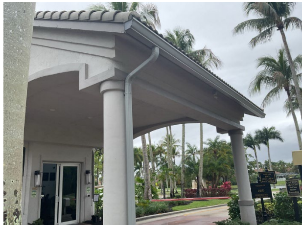
Aluminum gutters and downspouts
