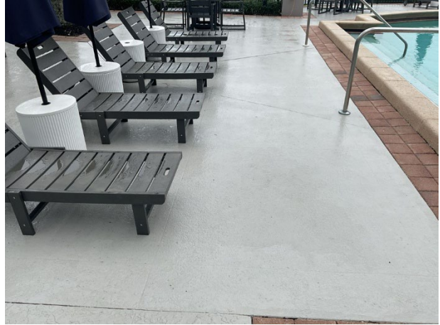
Concrete pool deck overview
