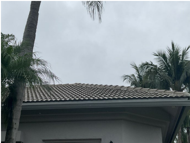
Concrete tile roof at clubhouse
