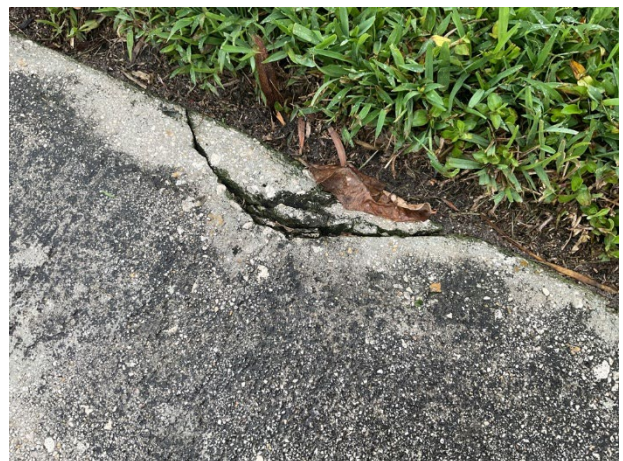
Sidewalk cracks
