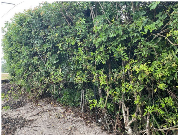
Chain link fence
