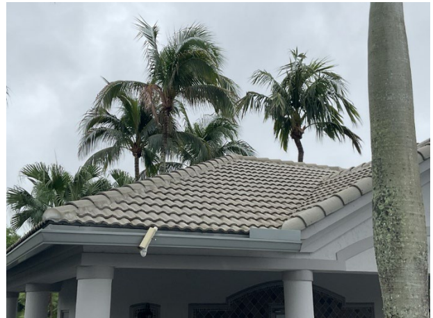
Concrete tile roof at pool house
