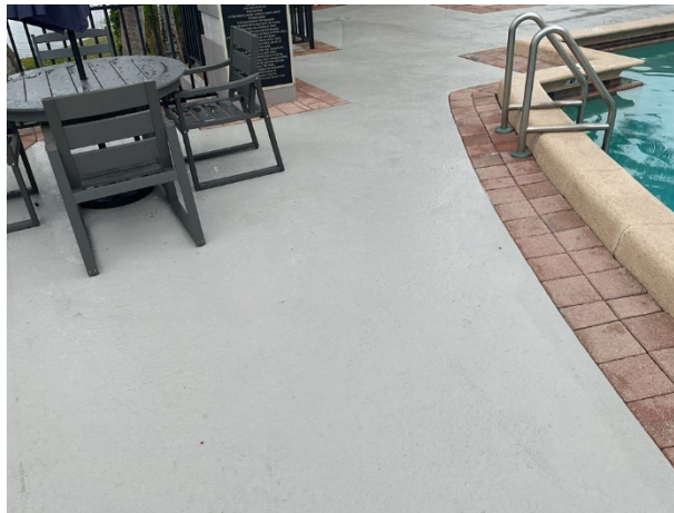
Concrete pool deck overview
