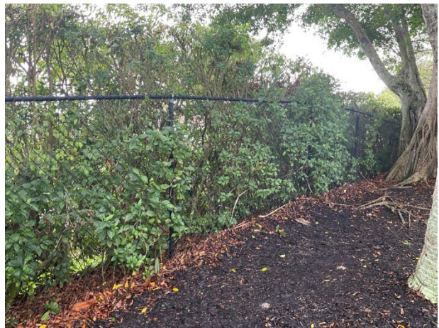
Chain link fence
