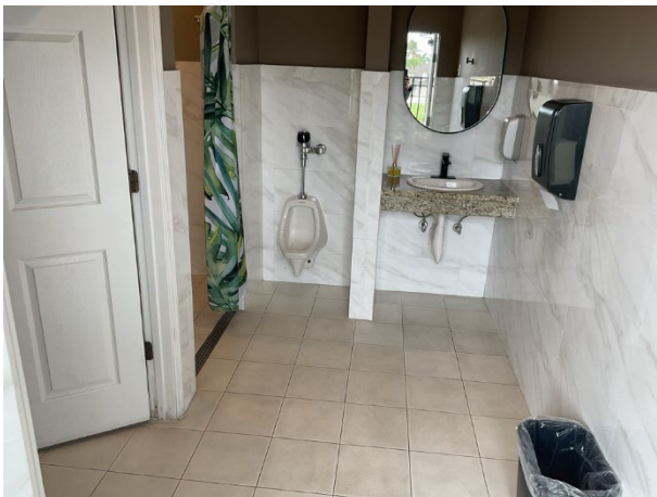
Pool house rest room overview
