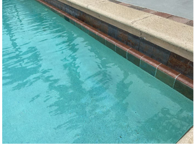
Pool plaster finish with tile perimeter
