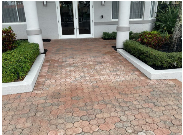
Pavers at pool area
