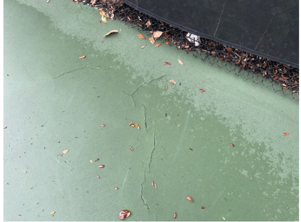
Surface cracks
