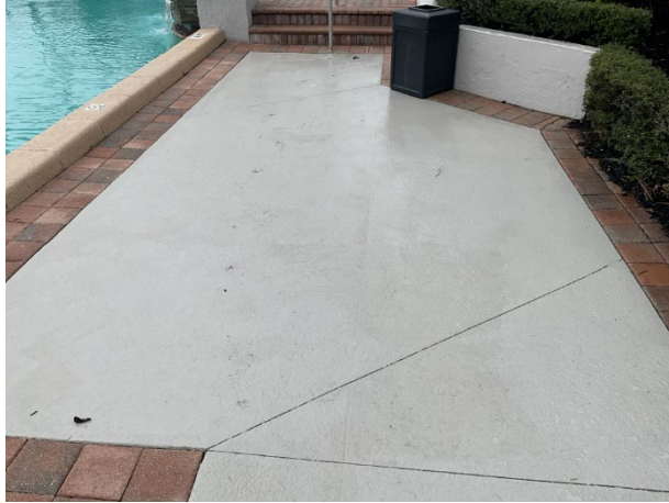
Concrete pool deck overview
