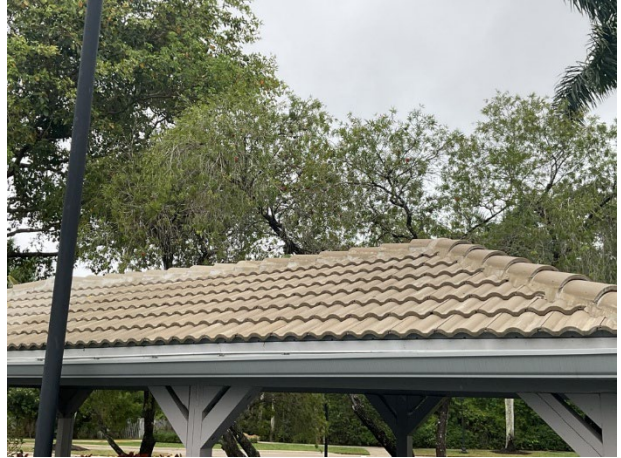
Concrete tile roof at tennis gazebo
