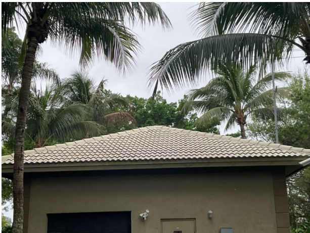
Concrete tile roof at maintenance building
