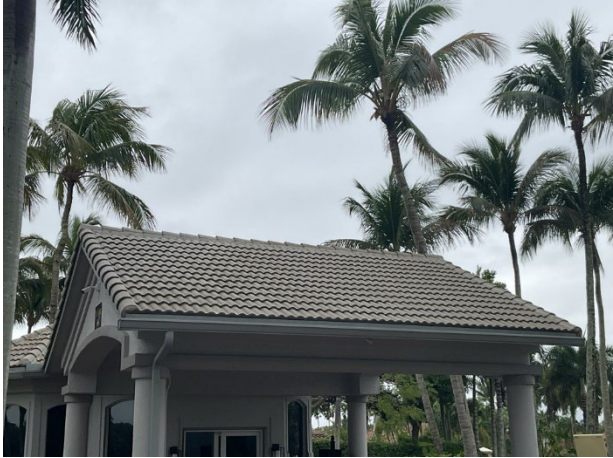
Concrete tile roof at guardhouse
