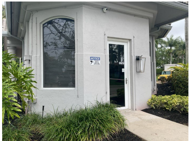
Common windows and doors
