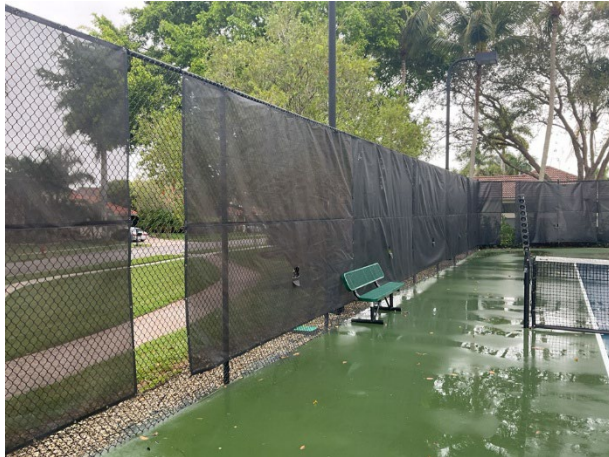
Chain link fence
