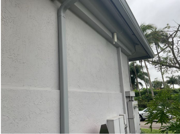
Stucco wall finishes
