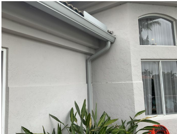
Aluminum gutters and downspouts
