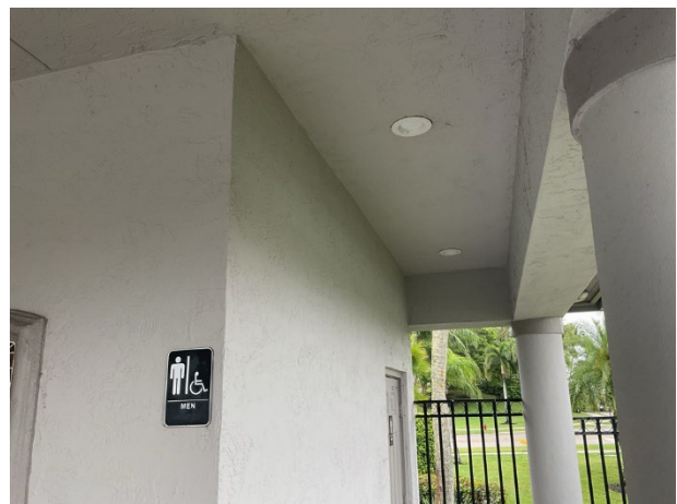
Stucco wall finishes
