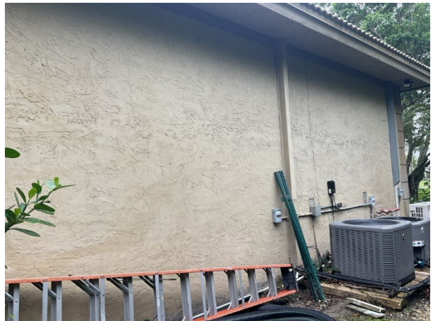
Stucco wall finishes
