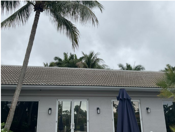
Concrete tile roof at clubhouse
