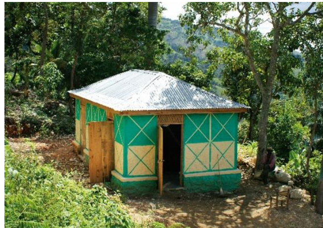
House in Haiti built with timber structure and stone filling and with a pitched roof. CRAterre
