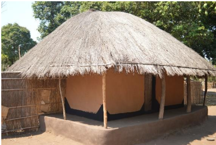
House built on a mound with adobe bricks walls and thatch pitched roof in Mpale, Mangochi, Malawi. Jon Twingi
