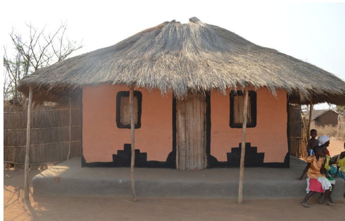
Decorated house with regular form and openings, thatched lightweight roof and four sides veranda (Malaza, Salima). © Jon Twingi
