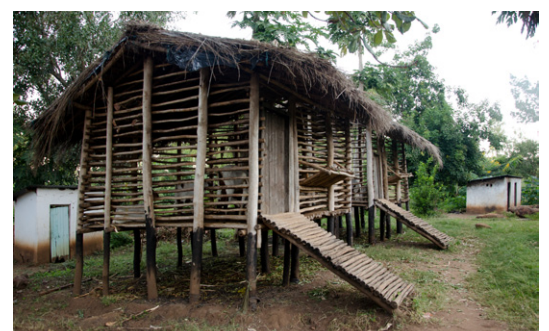
Raised constructions help protect small animals like goats or chicken from floods. These constructions are very common throughout the country. This is an example of raised goat pen at Naming'azi Farm Training Centre. CC- Carmichael C.
