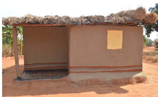
Thatched roofs are repaired when necessary. This house in Chome (Rumphi) presents thatch bundles which can be easily replaced when they get rotten. © Jon Twingi
