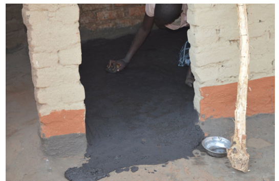
In some zones (e.g. Chaima, Dowa), used battery cells are cut and added to the mixture for earth floors. This can be a good practice regarding durability of plasters, but should be analysed also in regard to the health issues that it may cause. © Jon Twingi
