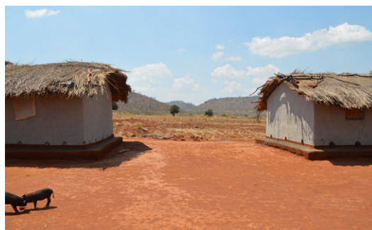
Distance between buildings is a good strategy to fight against the spread of fires. Most constructions in rural family homesteads are placed separately ones from the others. Homestead in Gausi, Nzimba. © Jon Twingi
