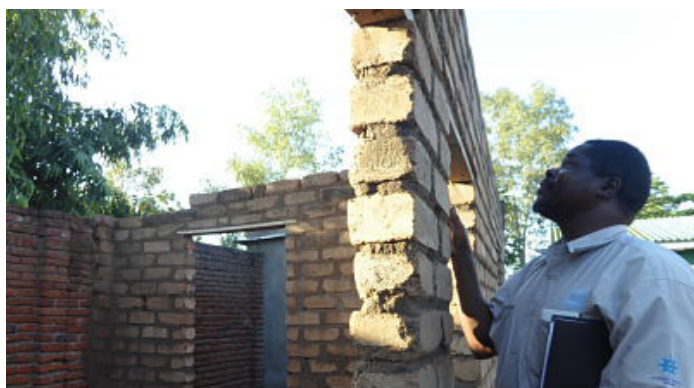
Walls with insufficient thickness and an important height are dangerous in the events of a disaster as they are not stable enough. CC- Ignacio Ngoma
