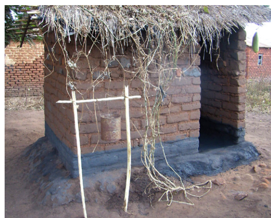
Hand-washing facility outside a pit latrine.
