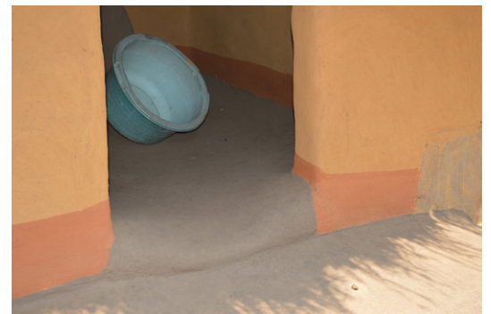
Well maintained earth floor in Chitungulu, Nkhata Bay. © Jon Twingi.
