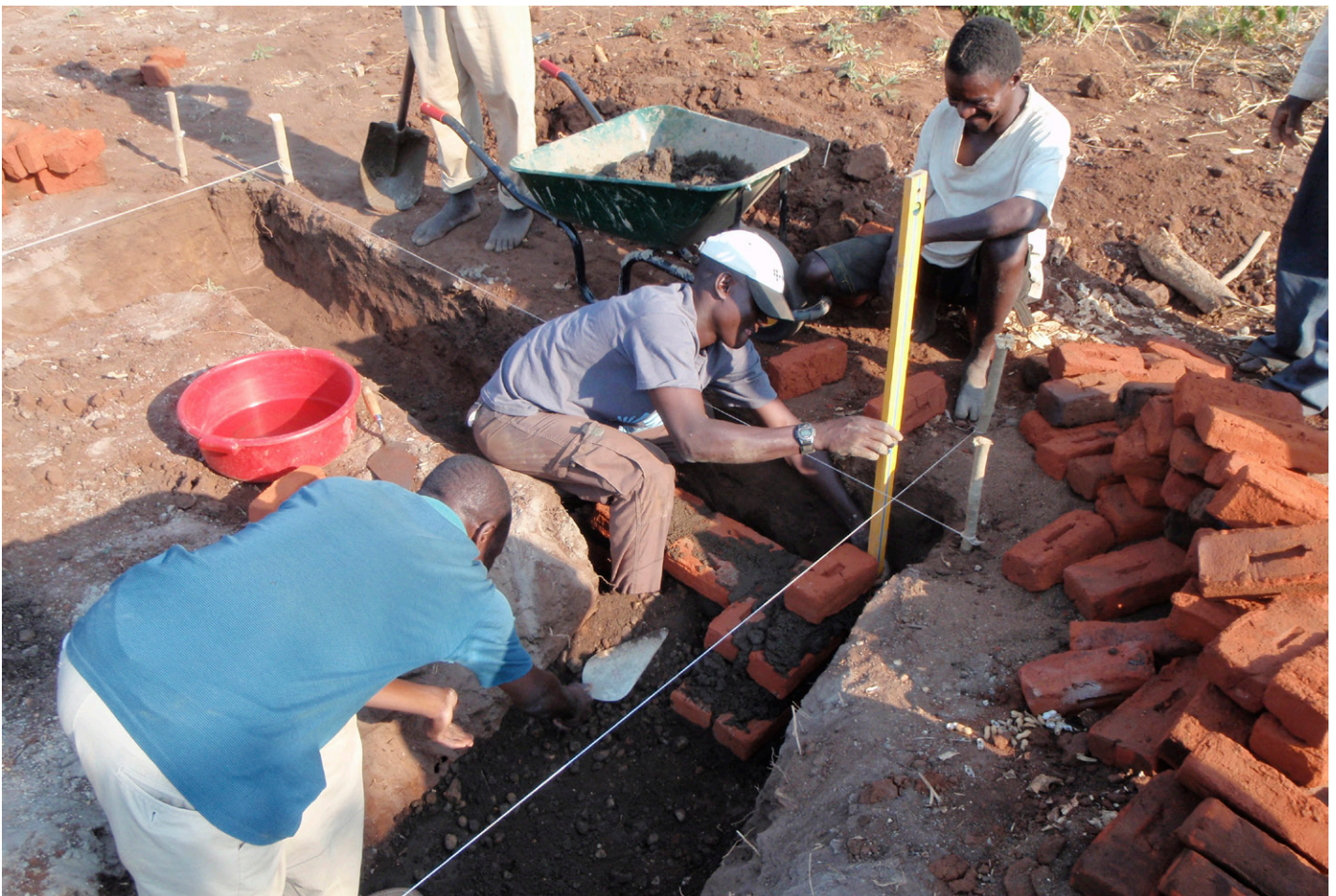
Construction of a foundation. CC- Gregory S.
