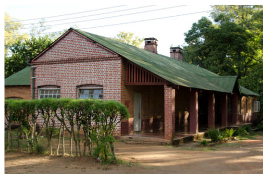
British colonialism also introduced in Malawi the use of fired red bricks, regular and paced windows and doors, concrete or burnt bricks lintels and roofs covered with corrugated iron sheets. Mission in building in Blantyre. CC- Carmichael C.
