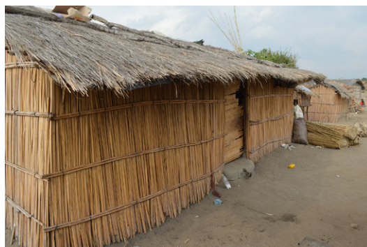
House built with timber or bamboo framework vegetal fibres in walls (reeds, bamboo) and roof (thatch).
