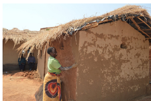
Woman plastering her house with earth plaster in Nkhombe, Kasungu. © Jon Twingi.
