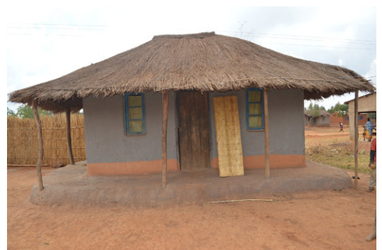
Main dwelling with four sides veranda in a compound in Kakhome, Dedza. © Jon Twingi
