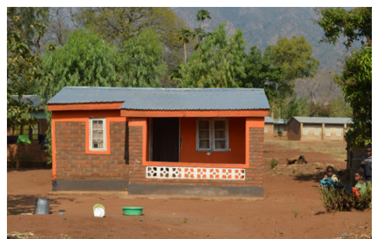
House with veranda built on a raised platform with burnt brick walls and gable roof covered with light metal sheets. Gawanani, Zomba. © Jon Twingi
