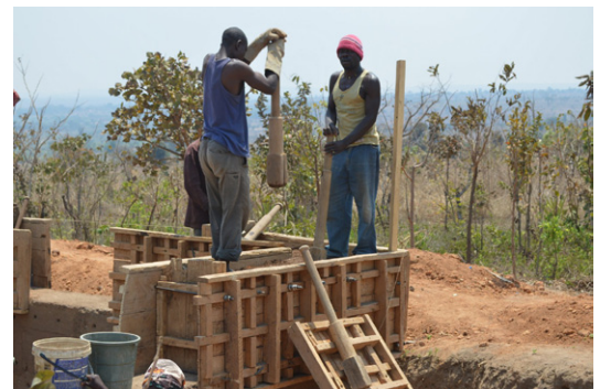
Many constructions in Malawi are built using local, renewable materials with little impact in the environment when they are well managed. This image shows the construction of a rammed earth house in Nisanje, Lilongwe. © Jon Twingi
