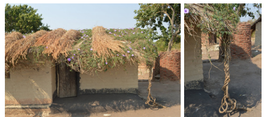
In some villages, the roof is used as a support for climbing plants. The risk of wrenching as well as partial or total uplift is reduced as the plants fasten together the roof components and attach the roof to the ground through the roots. House in Nsangu, Salima. © Jon Twingi
