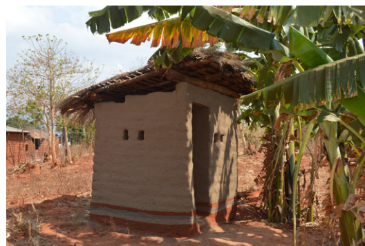
Latrine in Chome, Rumphu. © Jon Twingi
