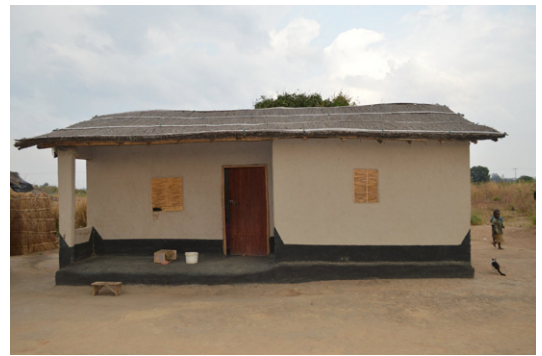
House built on a raised earthen platform with thatched gable roof and a plastering including colours for decoration and protection. Bisani, Nkhata Bay. © Jon Twingi
