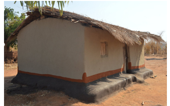
The earthen mounds are strengthened before the rainy season. The foundations are improved with an extra layer of mud. House in Chaima, Dowa District. © Jon Twingi
