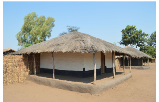
House with four sides veranda built on a raised earth platform with adobe walls and thatched hip roof. Chipile, Mangochi. © Jon Twingi
