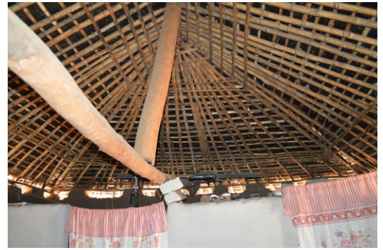
Bamboo is more and more used, for example in roof frameworks. Hipped roof in Dzipusile, Ntcheu. © Jon Twingi.
