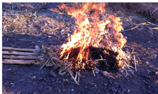
Timber poles are burnt to prevent termites' attacks before being inserted on the ground. Phalombe District. © CADECOM
