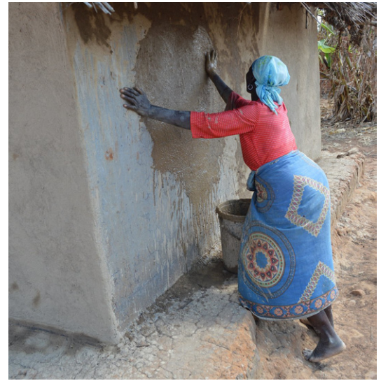
Women are involved in the construction, maintenance and protection of houses against particular hazards. Houses become more resilient thanks to this knowledge and know-how. Woman plastering in Chisi, Nzimba. © Jon Twingi
