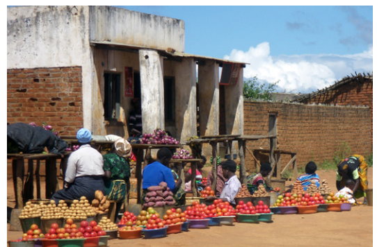
The roof of the veranda ( khonde ) is structurally independent from the main roof of the building in order to avoid damage to the main building roof during strong windstorms. Construction in Karonga. © Sonia Molina
