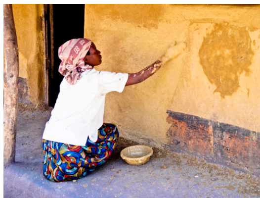
Woman cladding a wall with earth plaster. CC- Gregory S.
