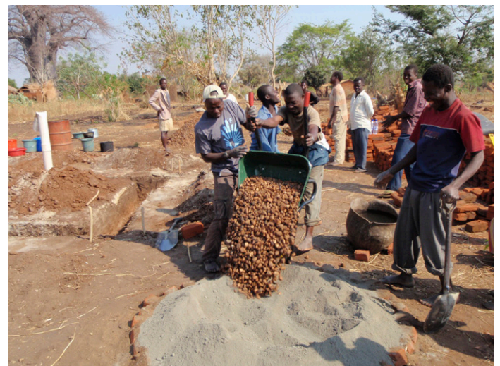
Stage of construction of foundations of a house.
