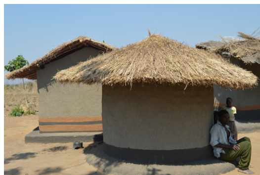
Round and rectangular plan constructions built on raised earth platforms in Juma, Dowa District.
