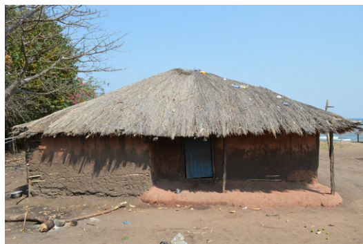
House with veranda built on a raised platform with wattle and daub walls and thatched hip roof. Mkwamwiyo, Karonga. © Jon Twingi
