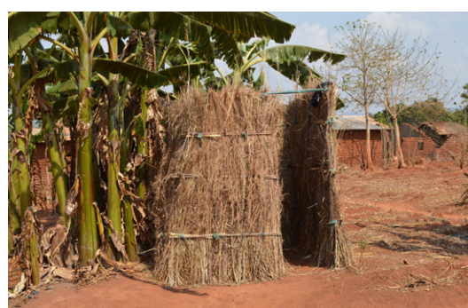
Latrines and showers are usually built using vegetal materials such as grass, timber, bamboo or reed. Latrine in Chome, Rumphu. © Jon Twingi
