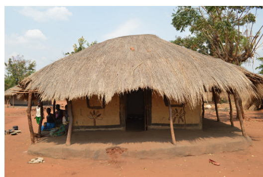
Verandas and large roof overhangs between the interior earth wall and the exterior avoid the risk that changes in humidity associated with rain will swell the soil under the walls. House in Simwaka, Nkhhotakota. © Jon Twingi
