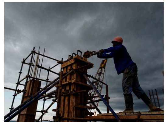
Reinforced concrete construction in Lilongwe. cc- ILO
