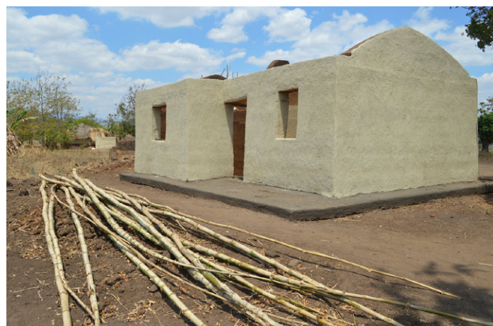
Rammed earth house under construction. © Jon Twingi
