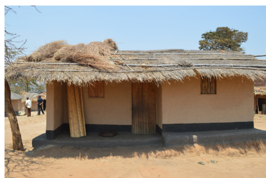
Longitudinal bamboo or timber pieces are sometimes joined to the roof's structure for better resistance to wind. House in Nyemba, Kasungu. © Jon Twingi
