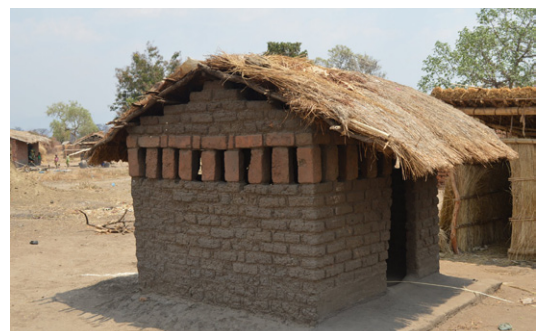
Small openings in the masonry walls allow adequate ventilation in the interior of the buildings, particularly in kitchens. Kitchen in Kalinyka, Ntcheu. © Jon Twingi
