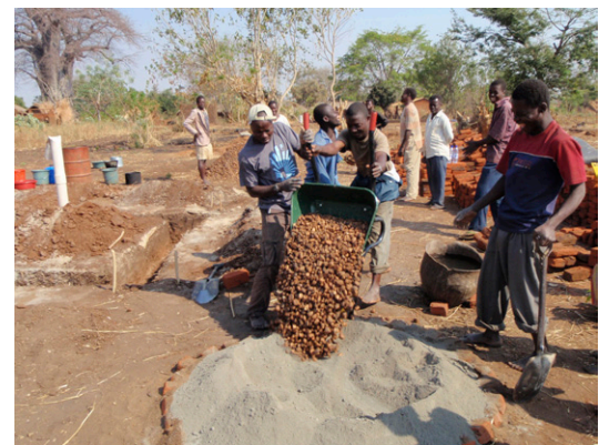
Mixing cement, sand and gravel for concrete. CC- Gregory S.
