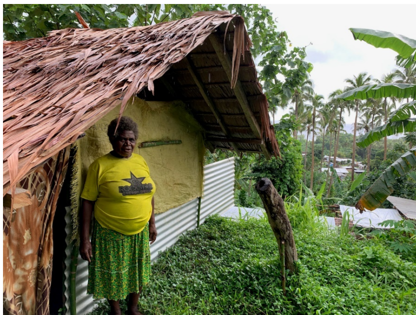
Fig. 4: An elderly widow in the Rangsuksuk community, Pentecost, who partially rebuilt her house after TC Harold with some support from CARE and her son. The natangora (sago palm) roof was built with salvaged leaves from the previous destroyed house together with some leaves supplied by CARE obtained from the neighbouring island of Maewo.
