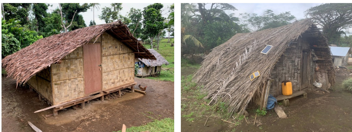
Fig. 6: A typical house in Pentecost (left) and in Tanna (right) built with natural materials.
