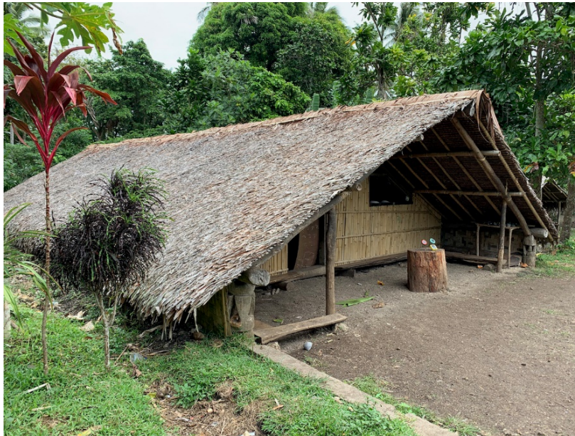
Fig. 7: A traditional safe house in the Merino community, Maewo, built after training on safe traditional construction.
