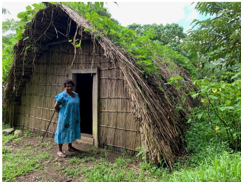
Fig. 9: A traditional safe house ( Nimilatan ) built after TC Pam by LRTC but needing repairs. People did not consider it safe enough for protection in a cyclone.
