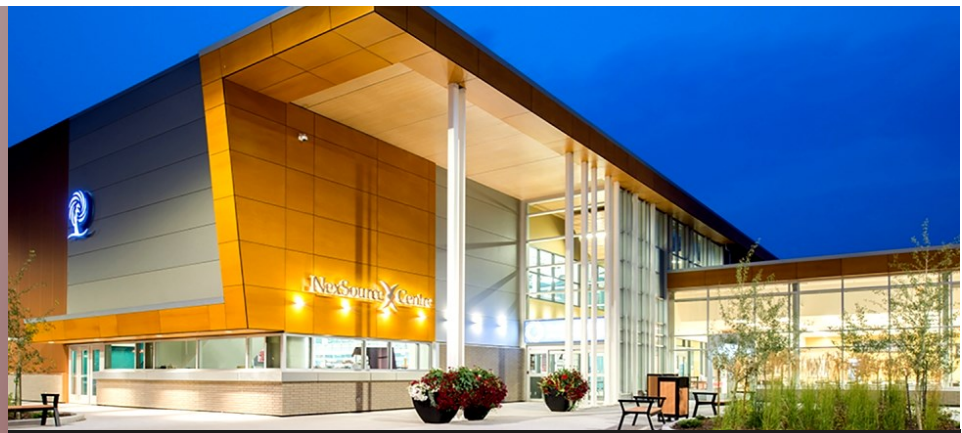
NexSource Centre, Sylvan Lake
