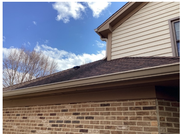
Weathered shingles (0N692 shown)
