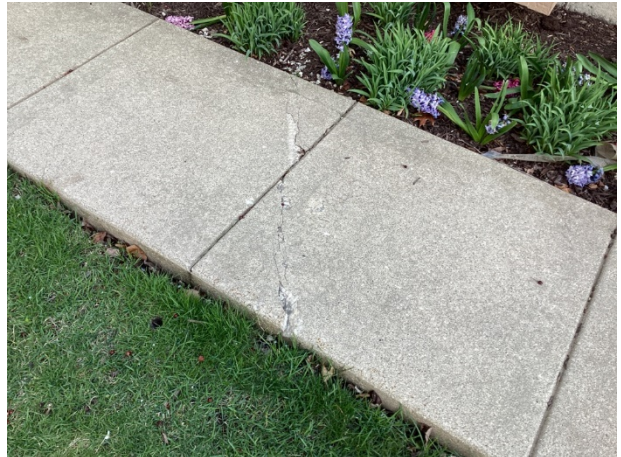
Sidewalk spalls
