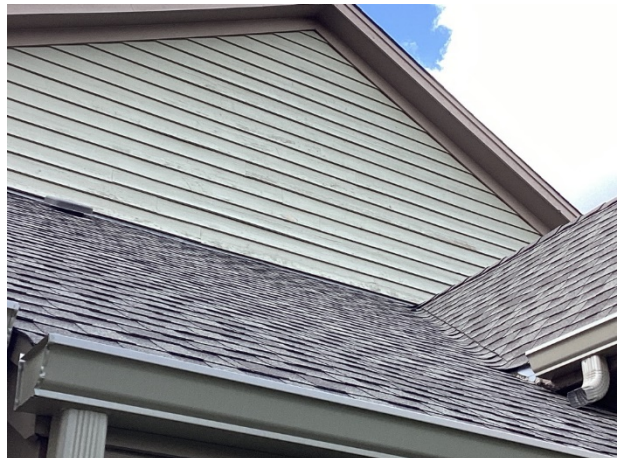
Siding deterioration
