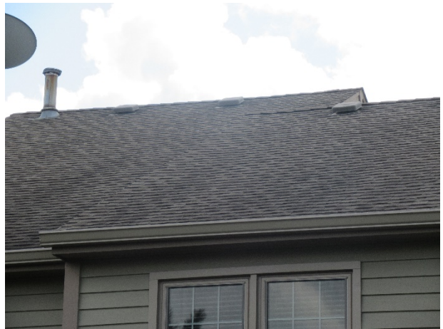
Weathered shingles
