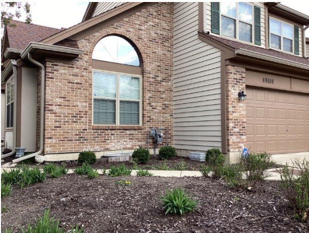
Masonry walls overview
