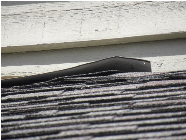
Flashing lift (0N665 shown)
