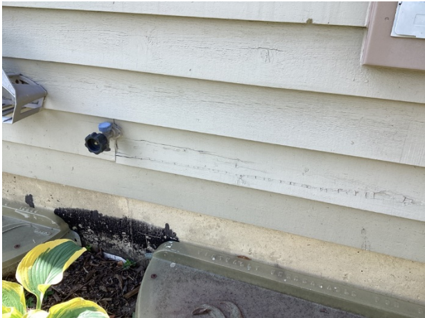
Siding deterioration
