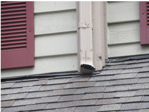
Downspout damage
