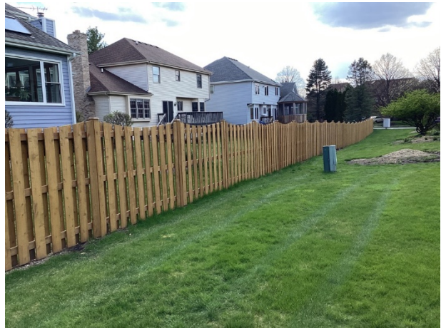
New fence section
