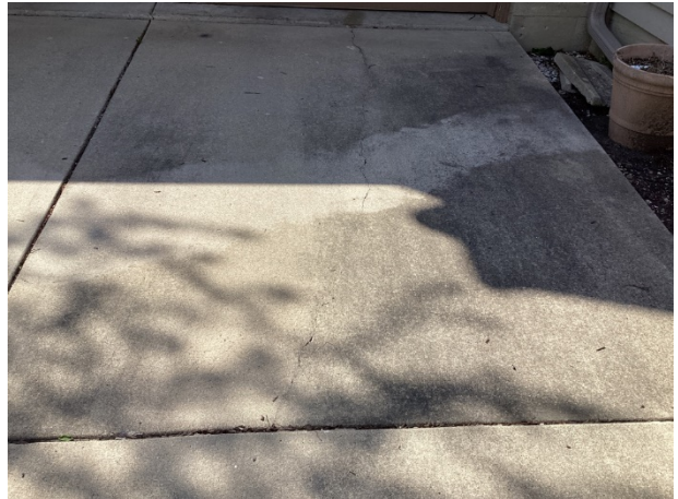
Driveway cracks
