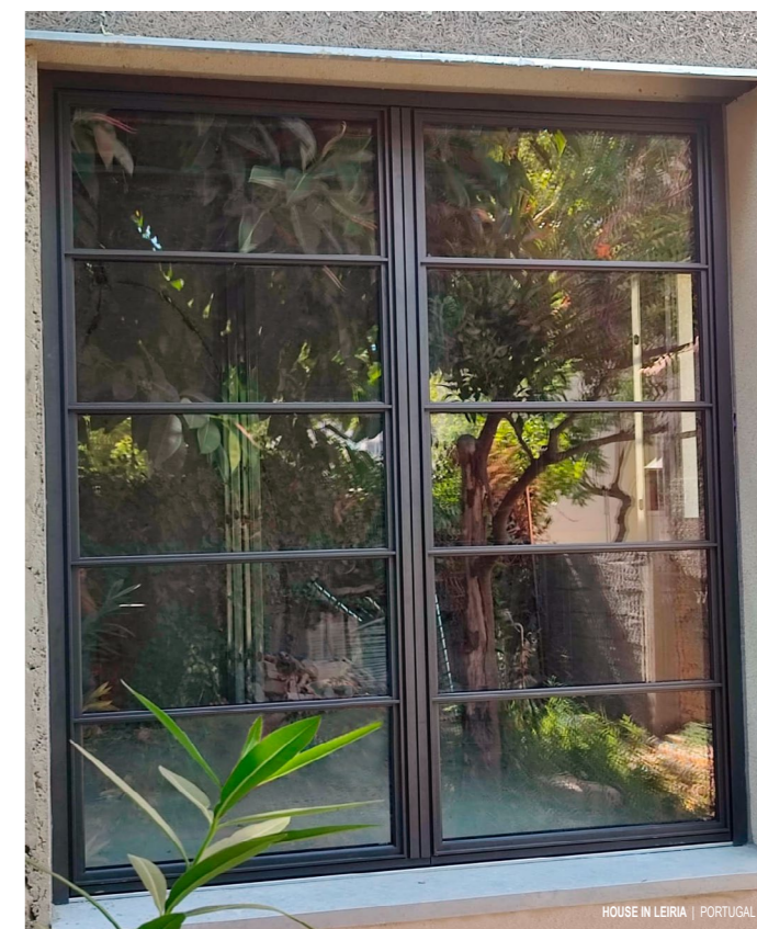
HOUSE IN LEIRIA | PORTUGAL
