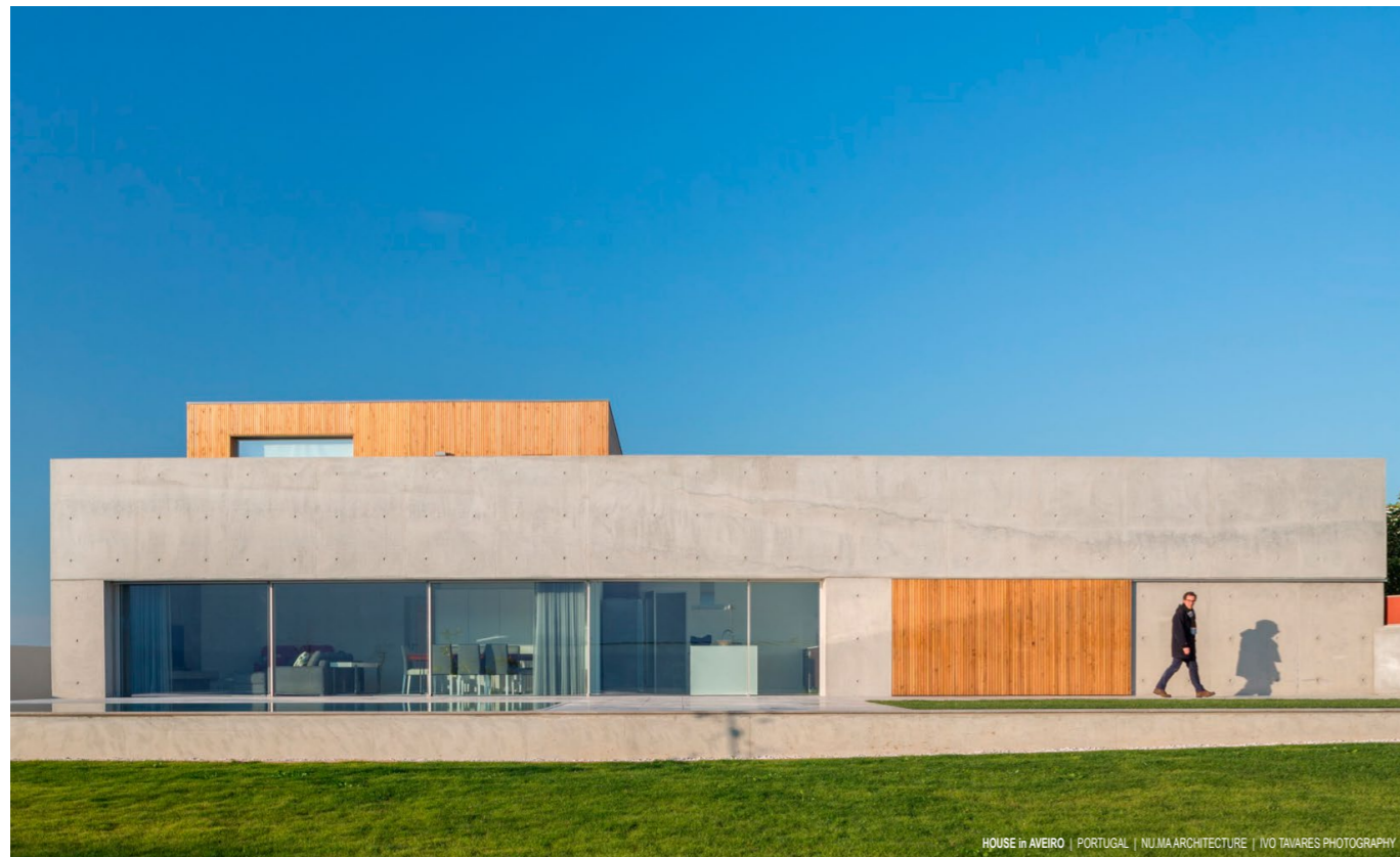
HOUSE in AVEIRO | PORTUGAL | NU.MA ARCHITECTURE | IVO TAVARES PHOTOGRAPHY
