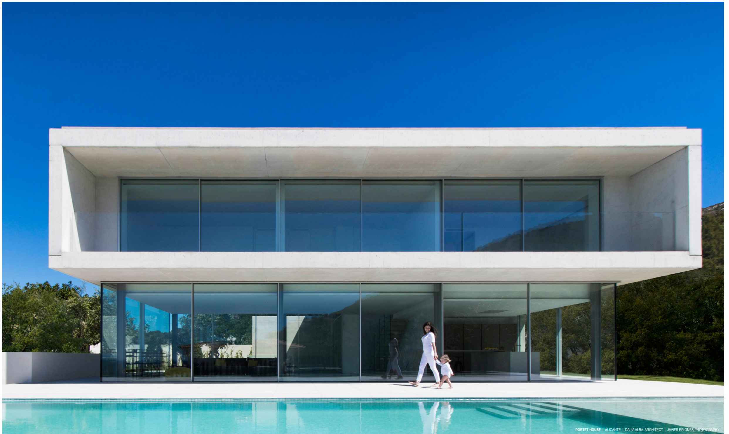
PORTET HOUSE | ALICANTE | DALIA ALBA ARCHITECT | JAVIER BRIONES PHOTOGRAPHY
