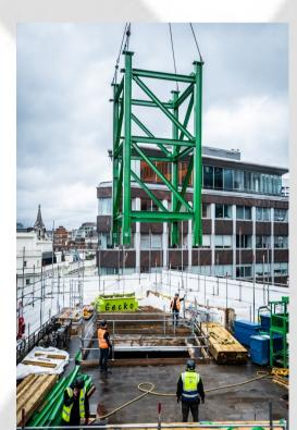
At the factory, the steel was shot blasted before refabrication to suit a new tower design, re-painted and assembled.
