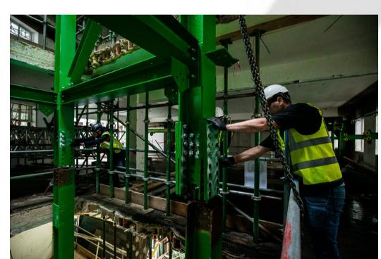
The refabricated tower was utilised on our Medius House site as a temporary support tower for the adjoining property.
