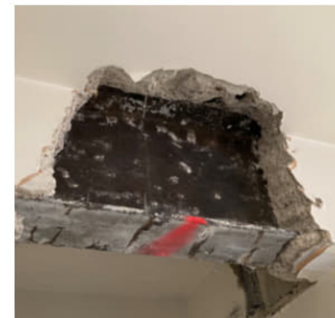
Phase 1 – Encasement removal in-situ
