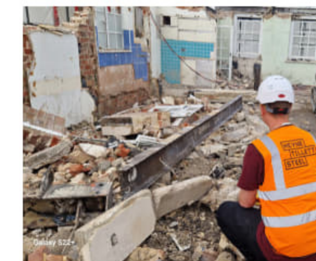
Phase 2 – Site photographs during deconstruction
