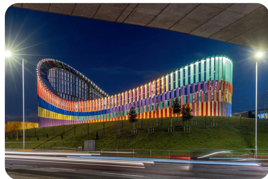
Early design team involvement meant that approximately 50% of the steel frame was sourced from re-purposed steel - 45 tonnes and 100 tonnes of embodied carbon saved
