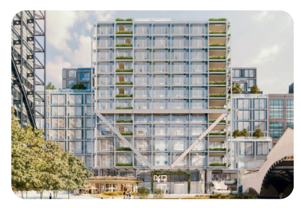
90% of the existing structure will be retained, having **50% lower embodied carbon** than a typical building of comparable size, with approximately **7,600 tonnes of embodied carbon saved**
