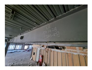
Pre-demolition survey and production of a steel inventory containing initial analysis of steel condition
