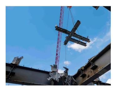
4 Craning steel sections for transportation to EMR testing facility
