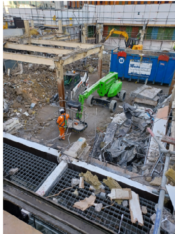
Cut and Remove Steel
