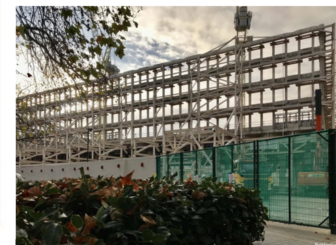
Steel from 30 Grosvenor Square Temporary Works
