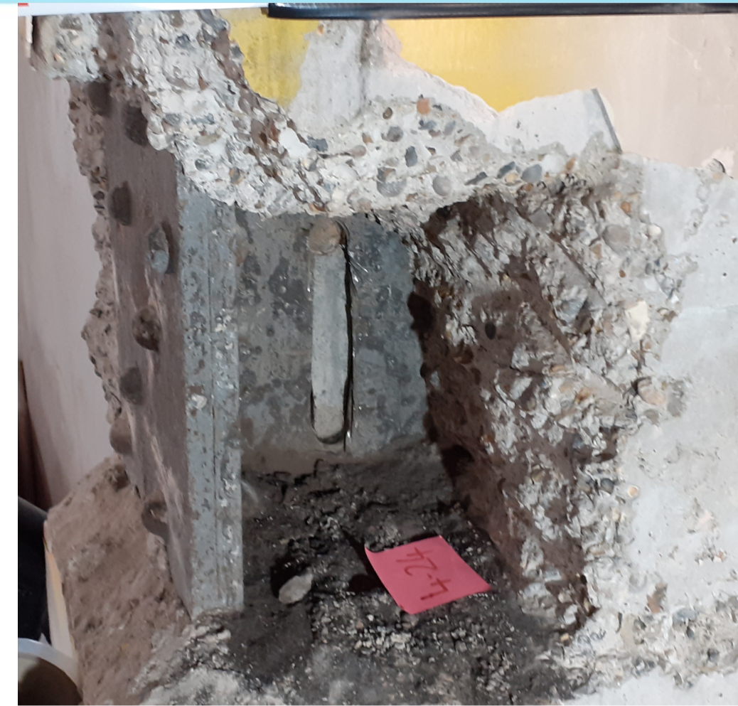
Initial sampling and testing of steelwork for design
