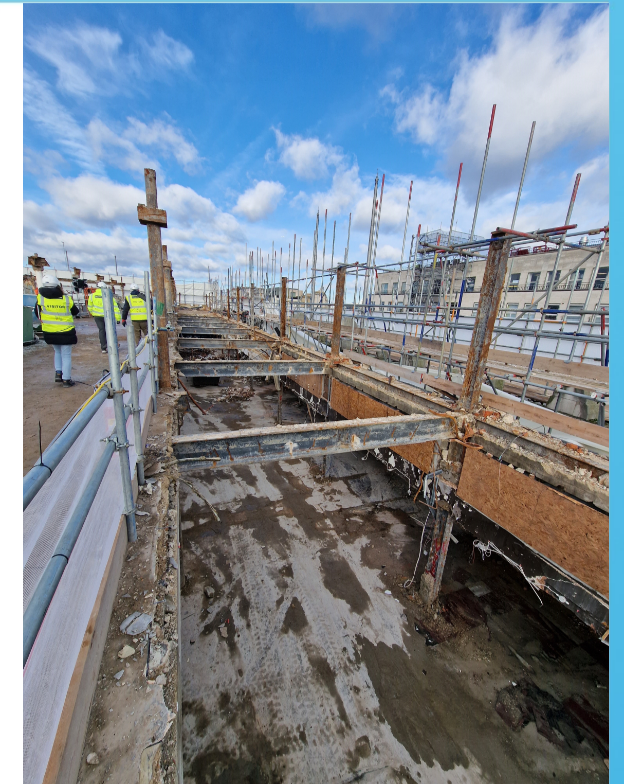
Members exposed and inspected on site
