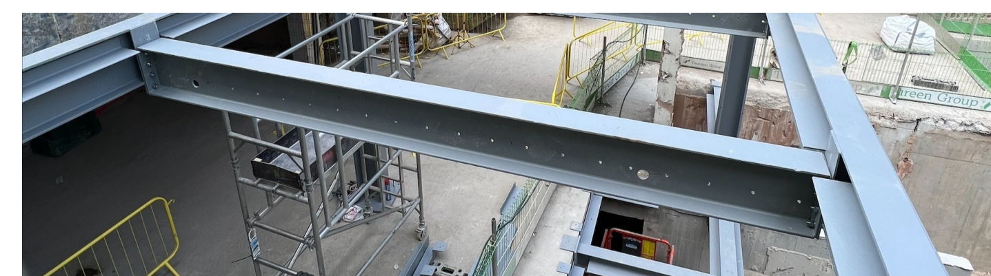
Refabricated steelwork erected on another site in London
