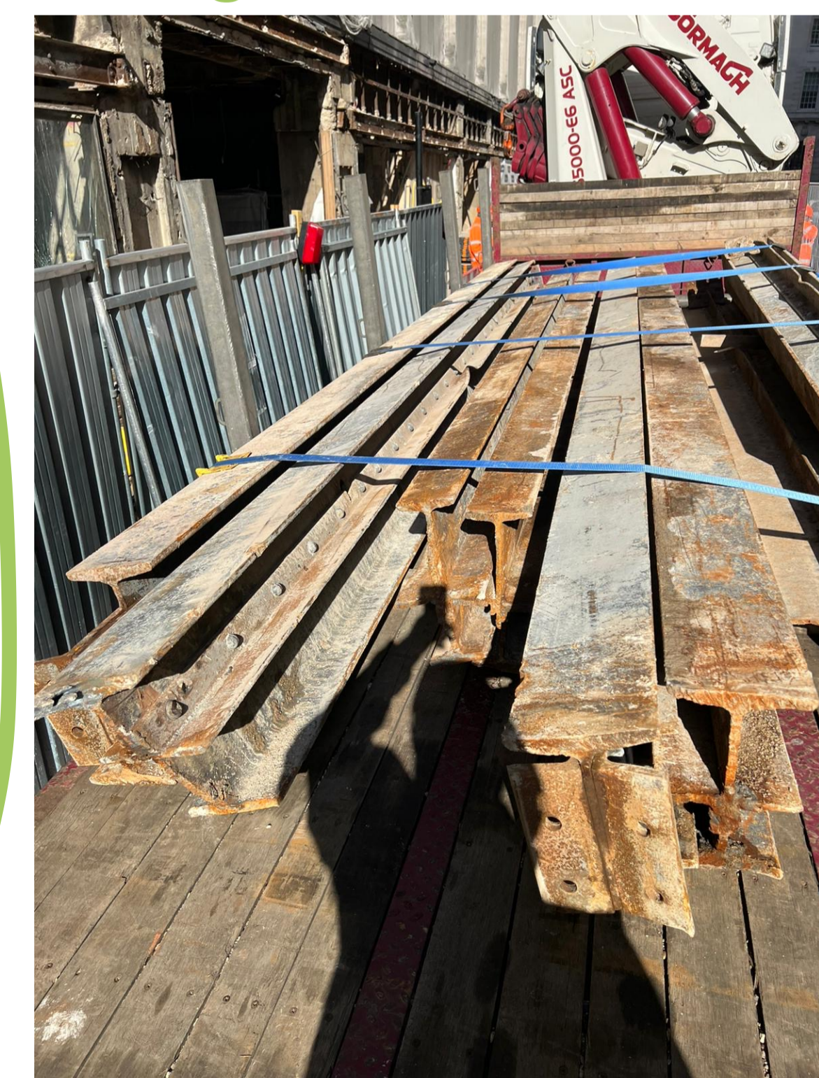
Steelwork sent for further testing and refabrication
