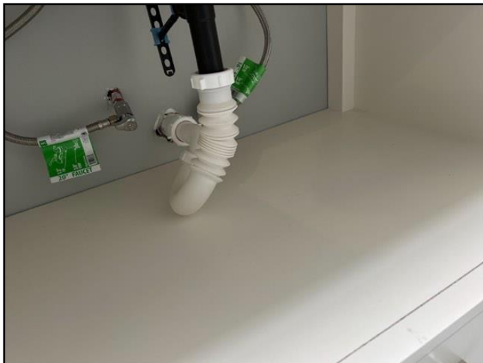
147. Flexible accordion waste piping
