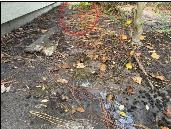
10. Ponding of water near ICV
