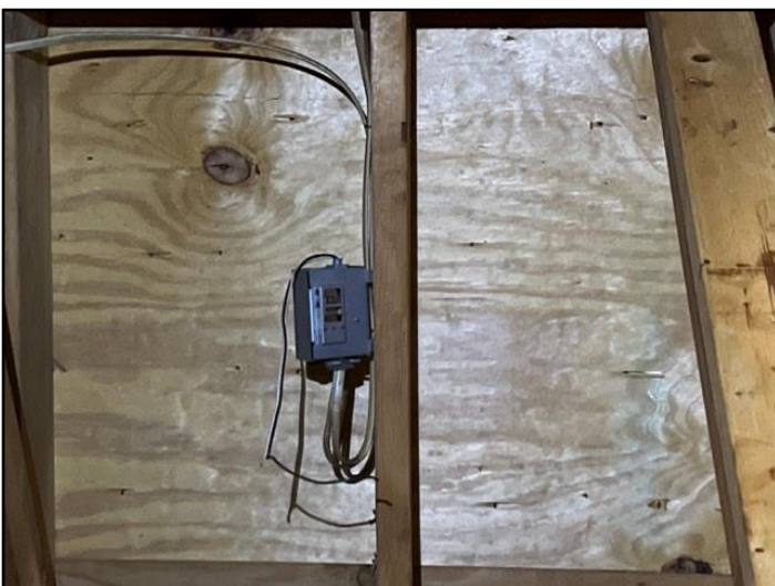
80. Exposed wires in attic
