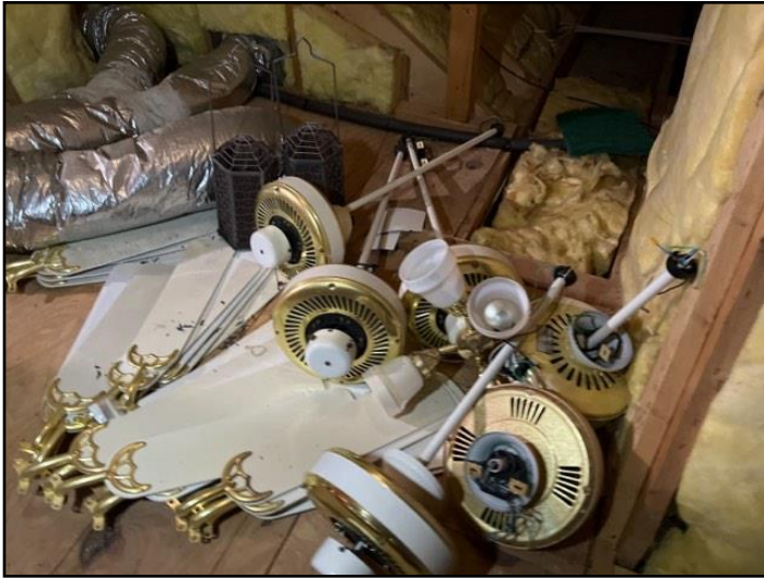
121. Debris in main attic
