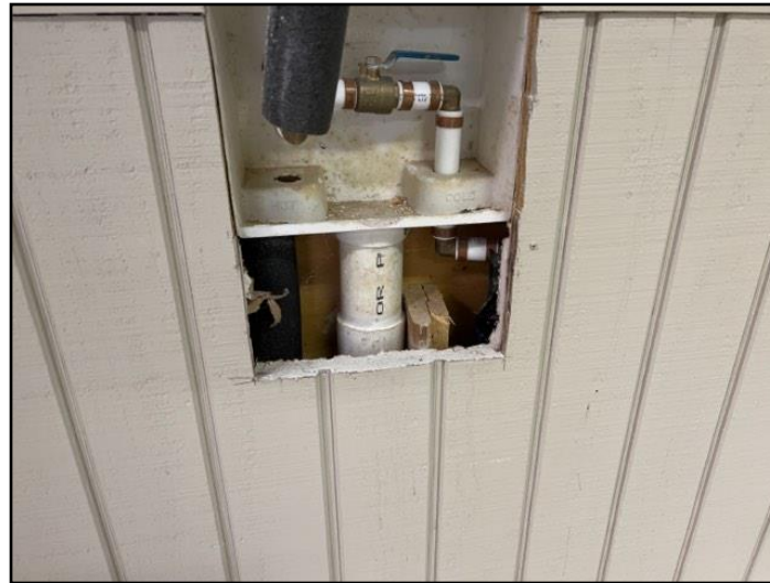
170. Open wall for access to plumbing
