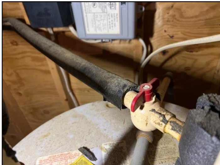
139. Water supply turned off
