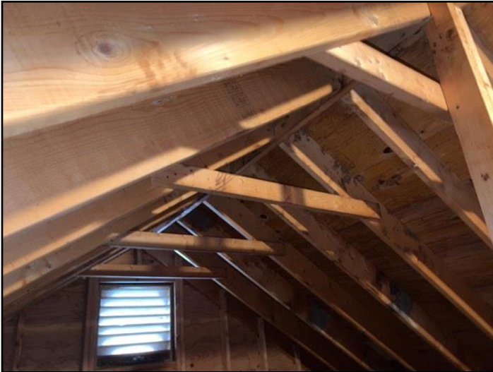
57. Rafters/ceiling joists garage attic
