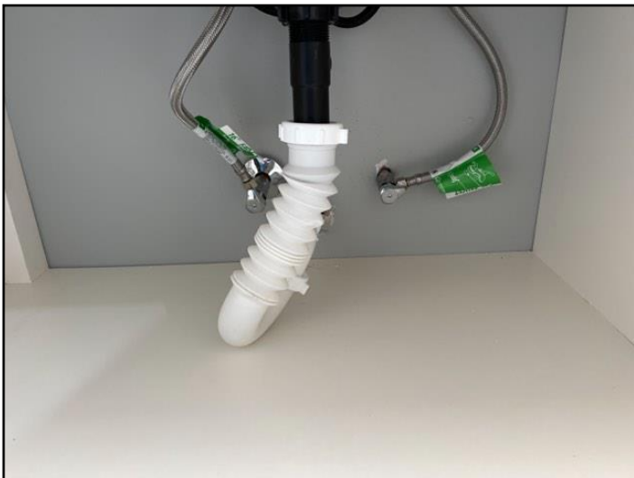
146. Flexible accordion waste piping
