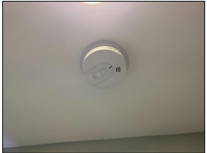
77. Ionization type Smoke alarm
