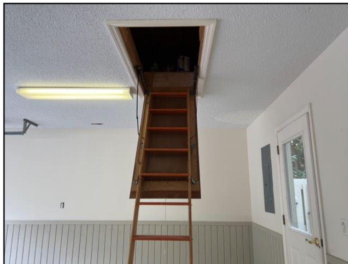
60. Pull down stairs in garage
