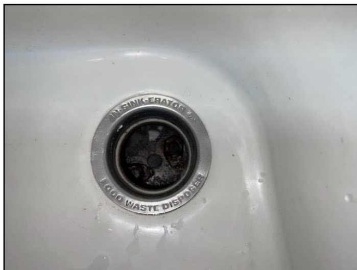
166. Splash guard missing
