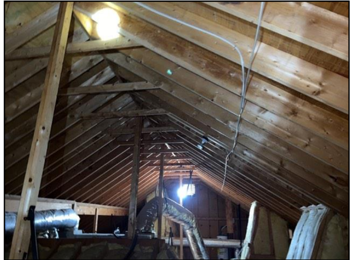
58. Rafters/ceiling joists, main attic
