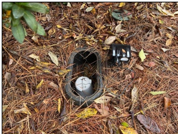
124. Meter on left side of property
