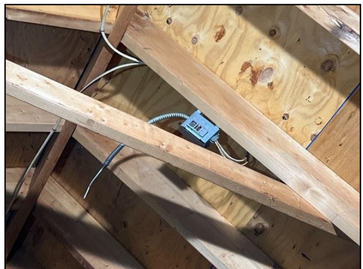
81. Exposed wires at junction box, attic
