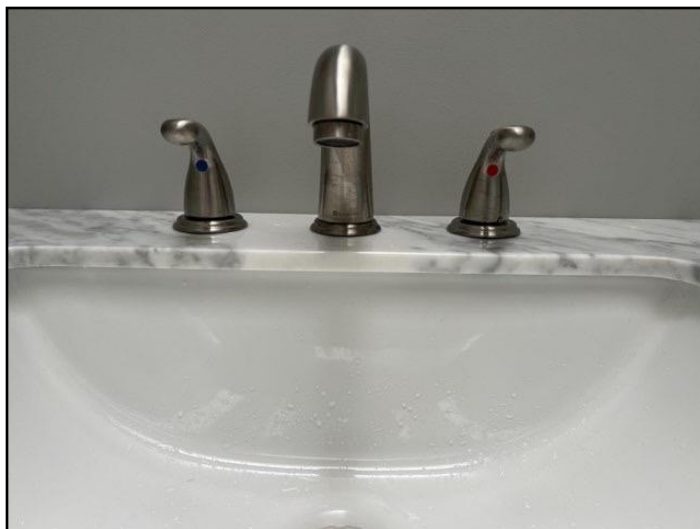
150. Hot and cold reversed, middle bathroom
