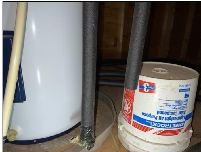
145. Cut supply piping
