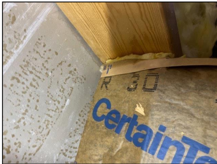
118. R-30 in attic
