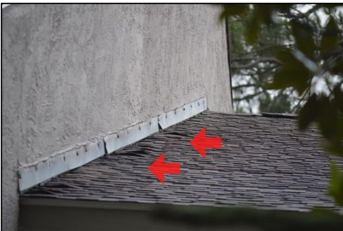
44. Damage, loose, open seams, patched
