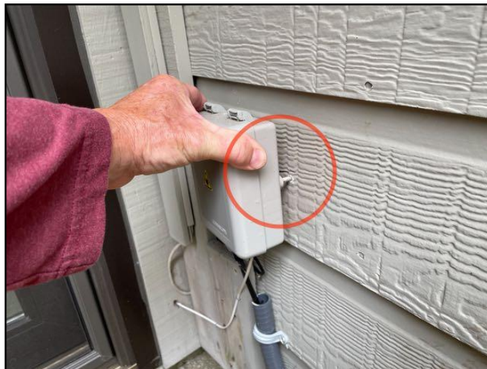
50. Cable Box loose on ext. wall
