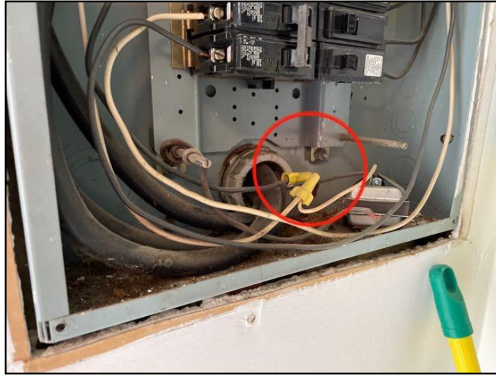
87. Neutral wire connect outside of bus bar
