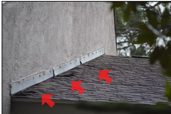
1. Bowing uplift of shingles
