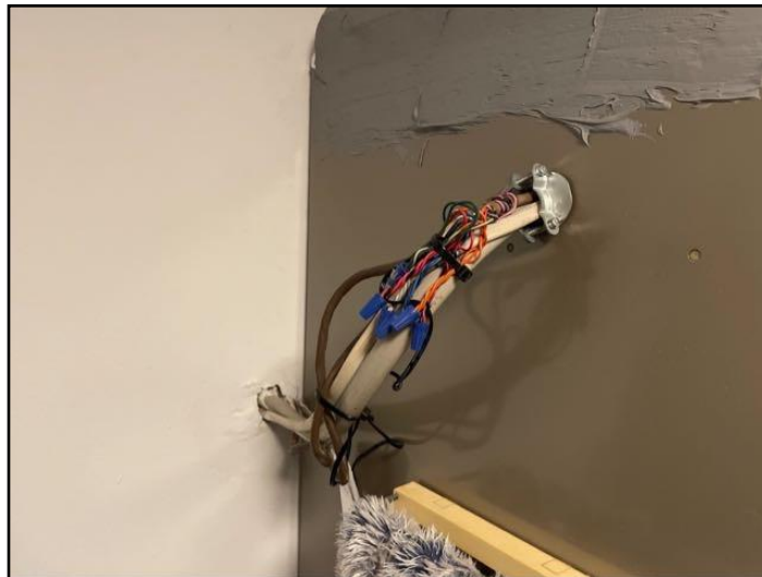
28. Open Splices Air Handler
