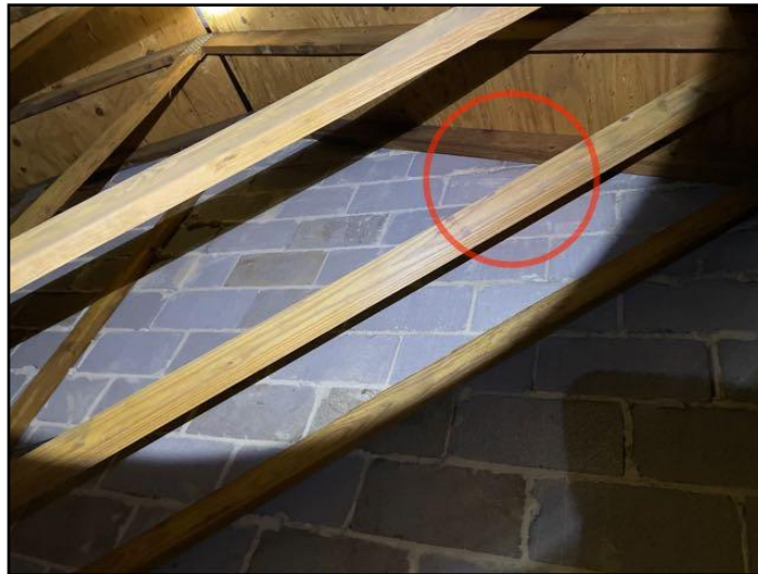
22. Ridge beam, Possible Water Damage
