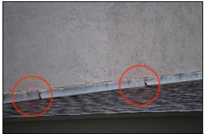
5. Open, loose seams Flashing
