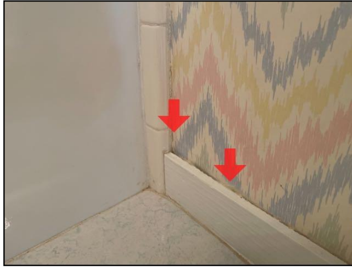
152. Possible Water damage
