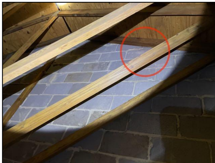
78. Ridge beam, Possible Water Damage
