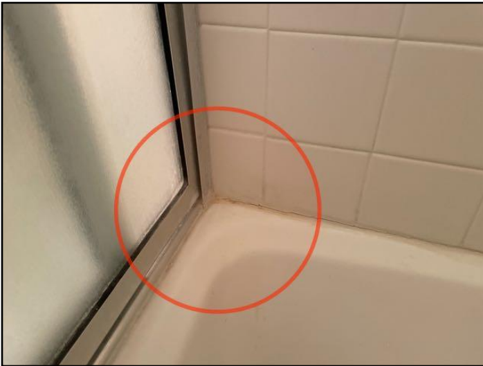
109. Grout loose, missing or deteriorated
