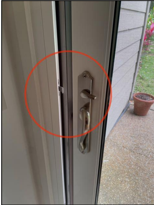
144. Lock not effective on exterior door
