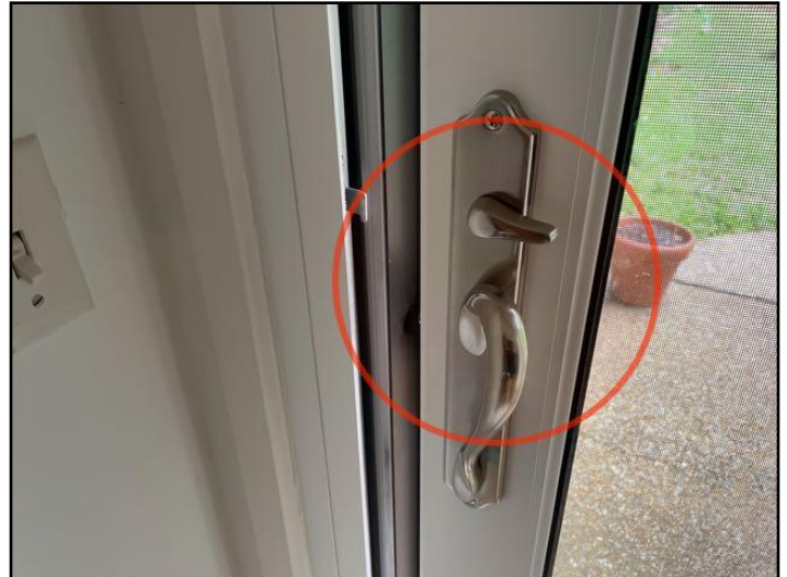
35. Lock not effective on exterior door
