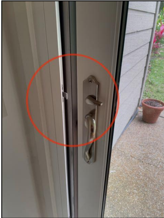
34. Lock not effective on exterior door
