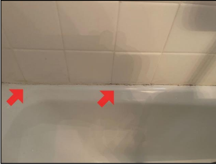
107. Caulking loose, missing or deteriorated
