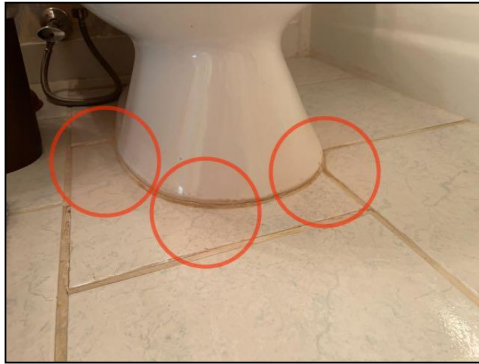
104. Caulking loose, missing or deteriorated
