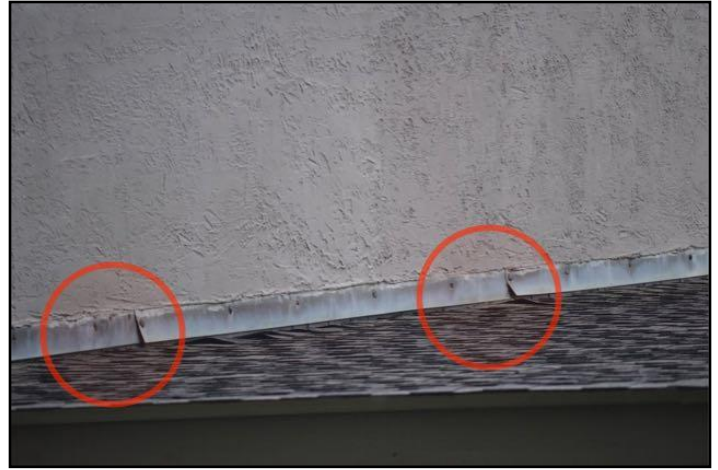
47. Open, loose seams Flashing
