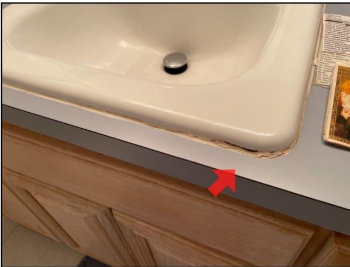
105. Caulking loose, missing or deteriorated
