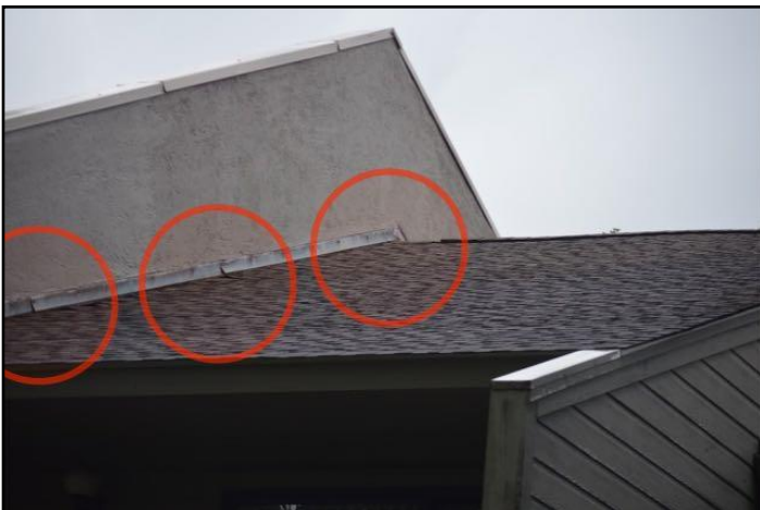
6. Open, loose seams Flashing
