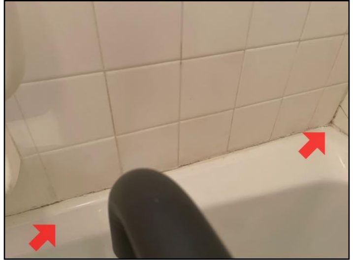
108. Caulking loose, missing or deteriorated
