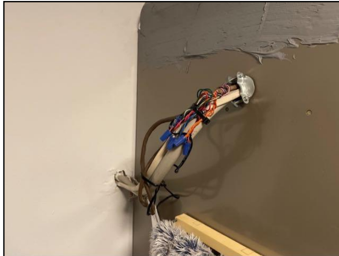
88. Open Splices Air Handler
