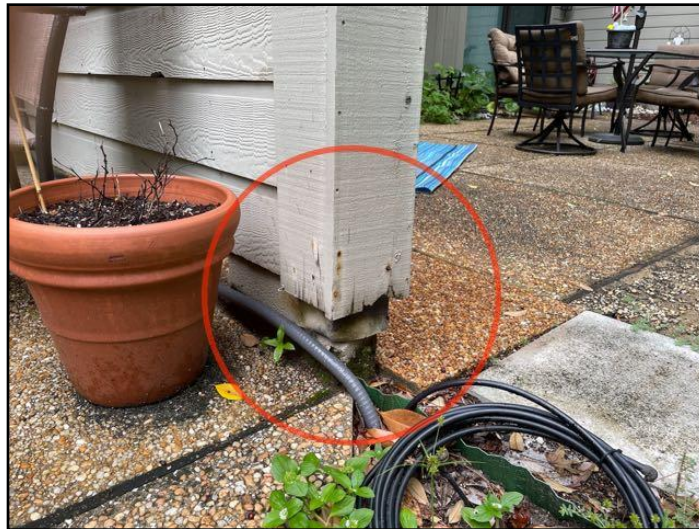
53. Rot or insect damage
