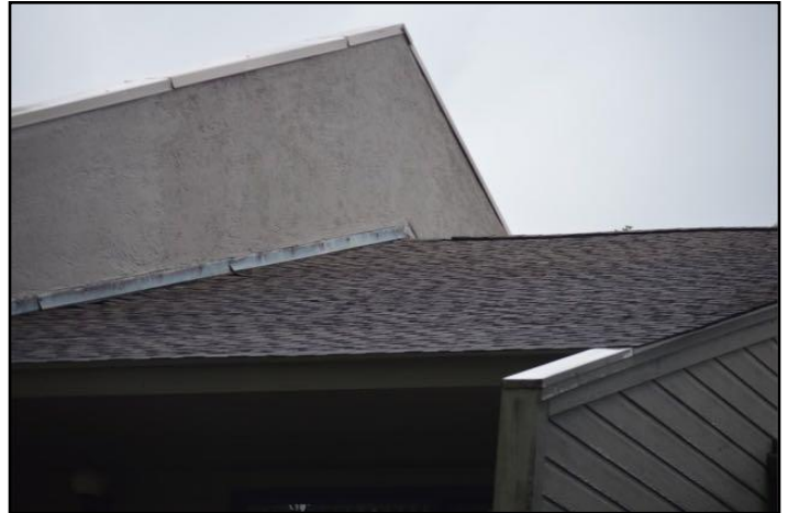
42. Asphalt Shingles
