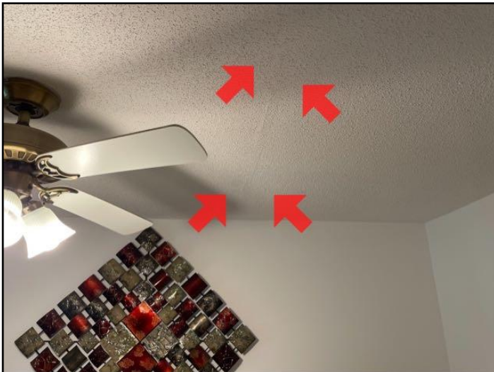
136. Tape on drywall Sagging
