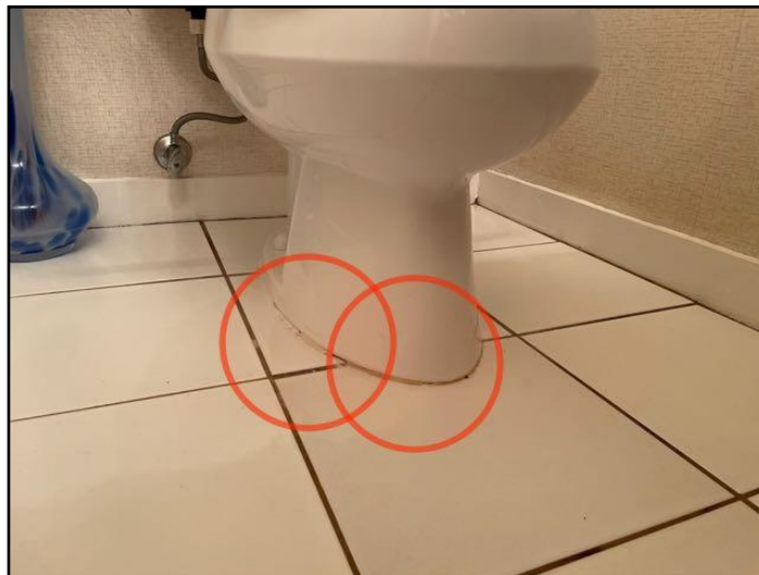
114. Grout loose, missing or deteriorated
