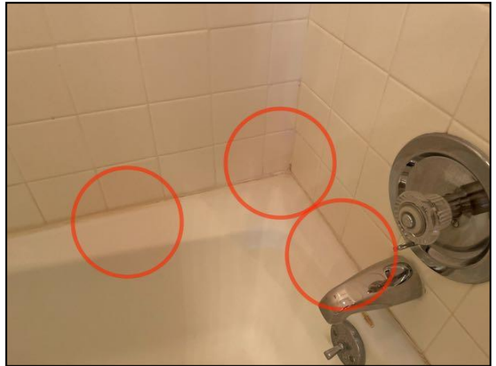
110. Grout loose, missing or deteriorated
