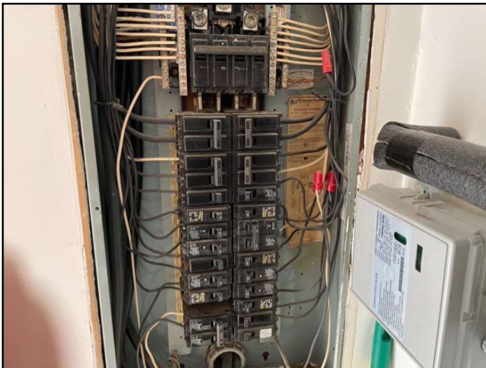
85. Wire nuts used in Panel
