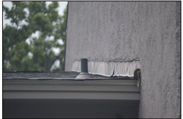
49. Loose open Seams Flashing
