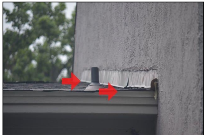
45. Open Loose Flashing
