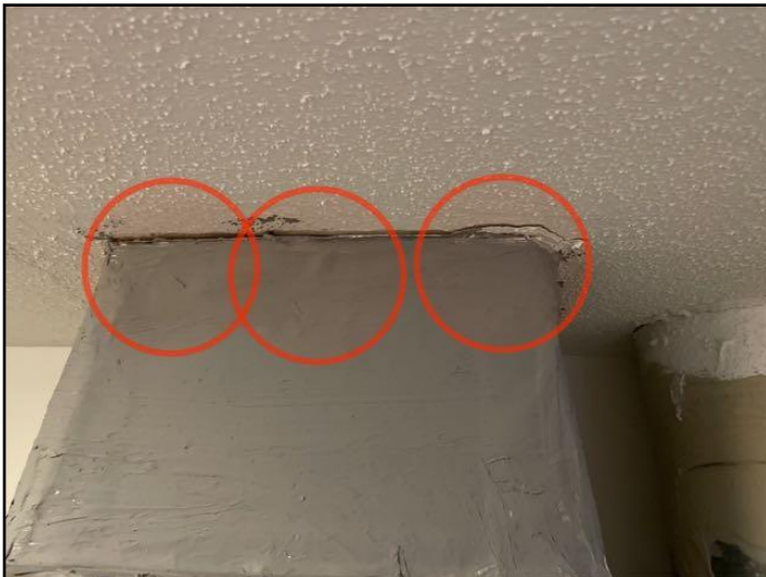
96. Loose/Missing Tape
