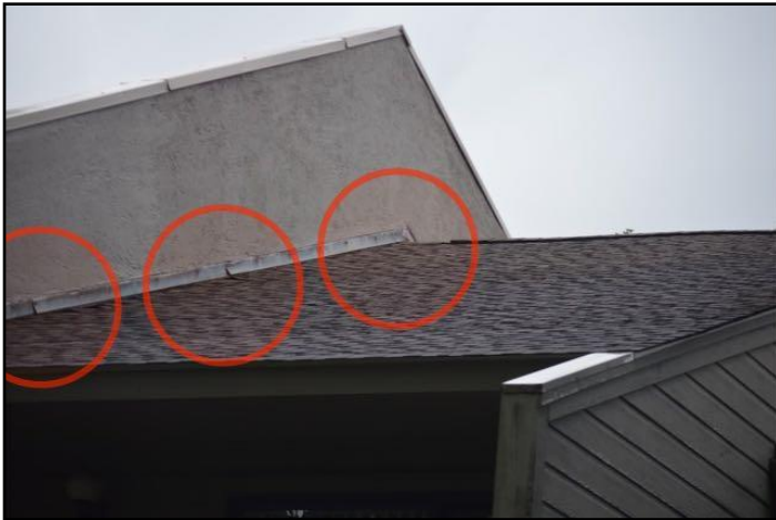
48. Open, loose seams Flashing
