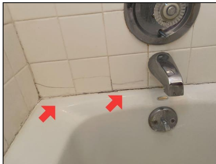
111. Tile loose, broken or missing
