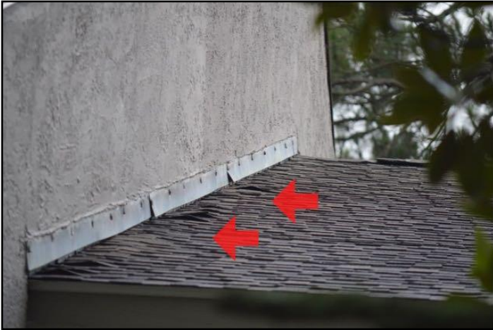
2. Damage, loose, open seams, patched
