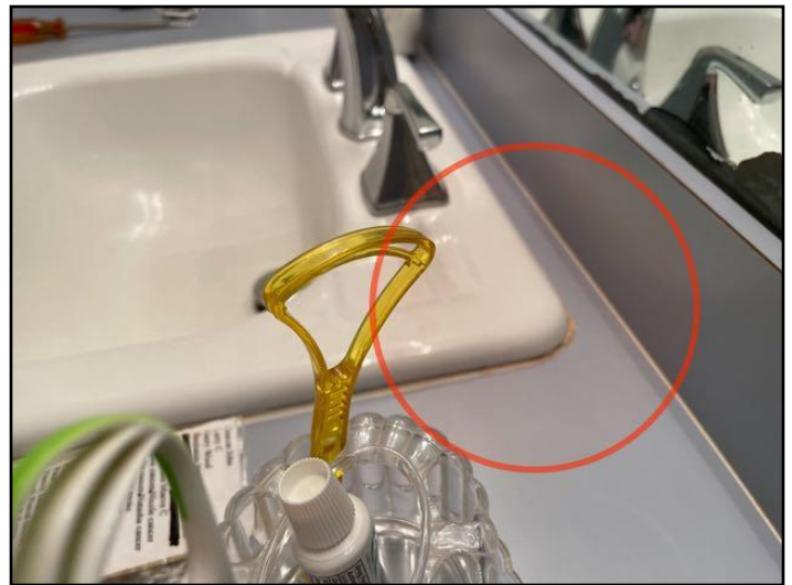
106. Caulking loose, missing or deteriorated
