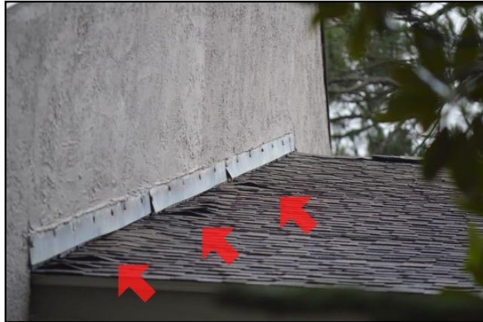
43. Bowing uplift of shingles
