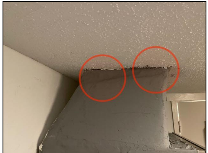
97. Loose/Missing Tape
