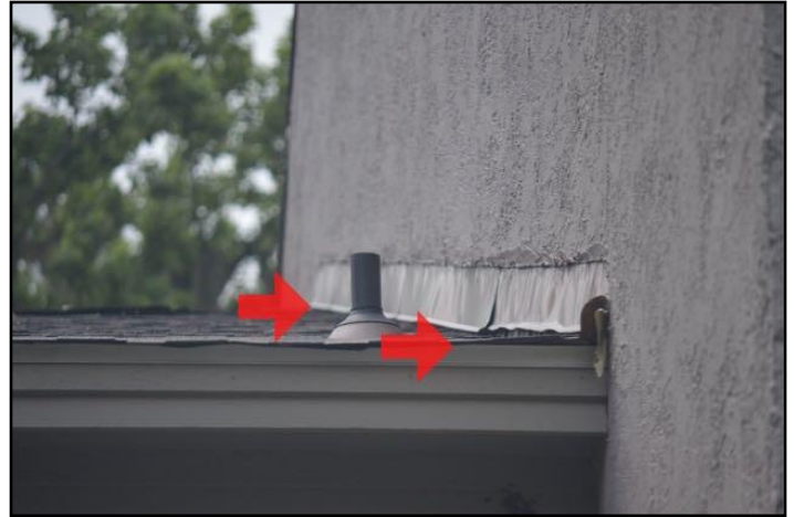
3. Open Loose Flashing
