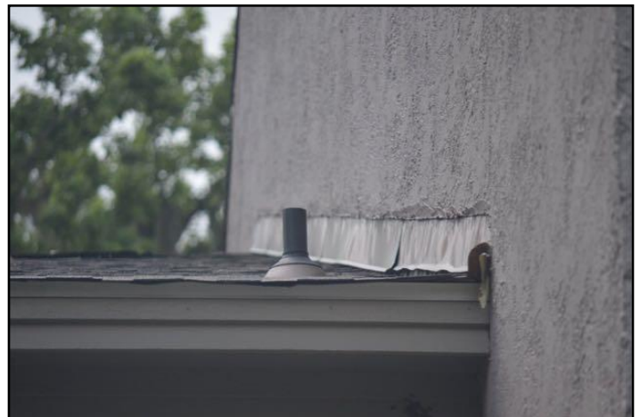
7. Loose open Seams Flashing
