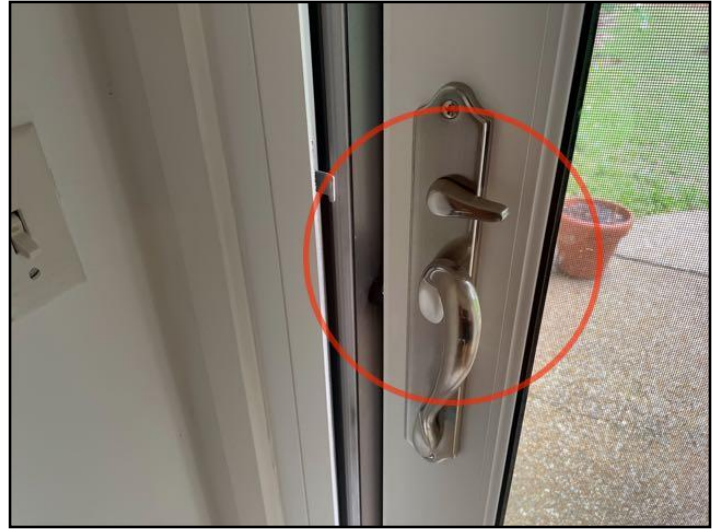
145. Lock not effective on exterior door
