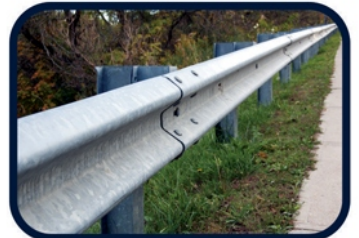
W Beam - Guard Rail
