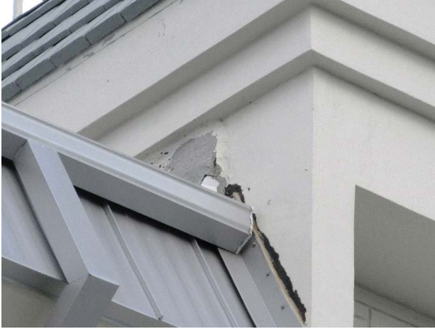
Coating finish deterioration
