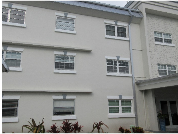
Metal gutter and downspout assembly
