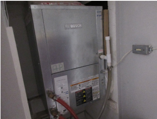
Lobby air handling unit heat pump overview
