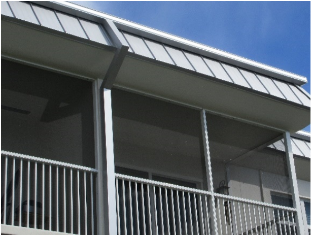
Metal gutter and downspout assembly
