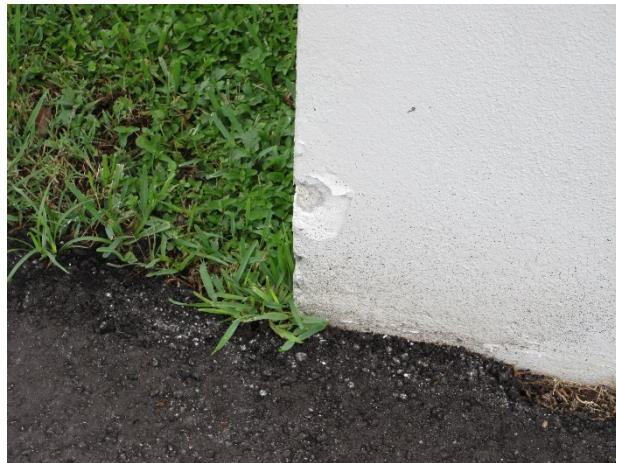
Coating finish deterioration
