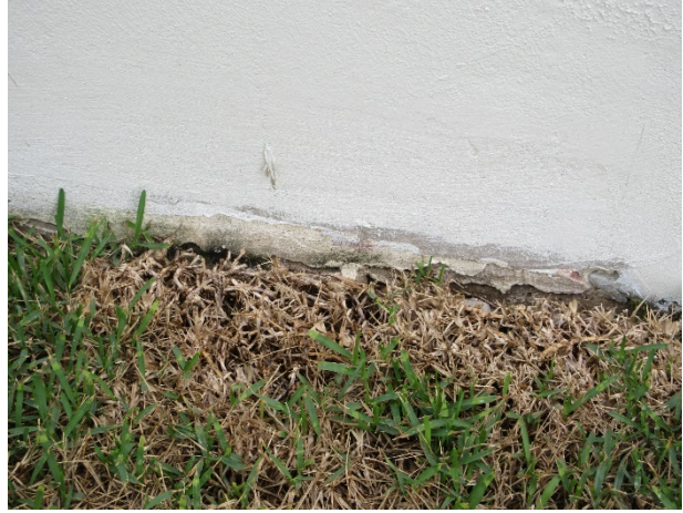
Coating finish deterioration
