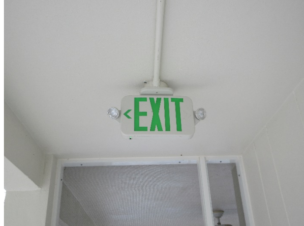
Life safety system emergency device
