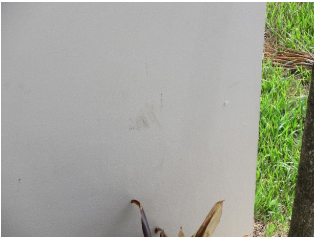
Coating finish deterioration
