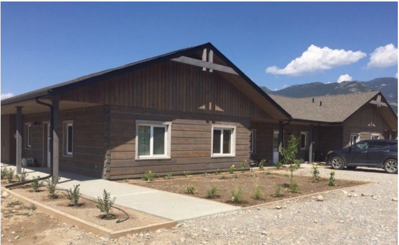
Outside with landscaping underway.
