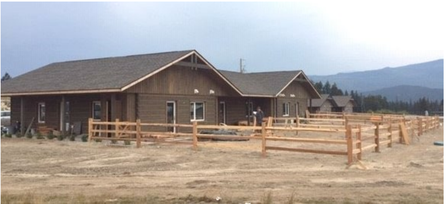
Rear view with fence under construction.
