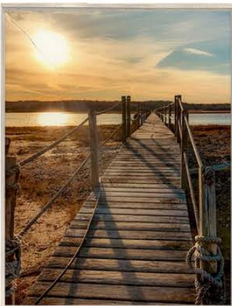
River Pier (JMA 2018)
