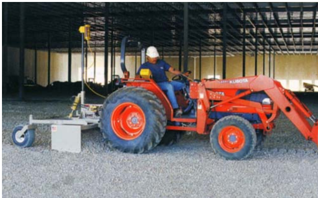
Laser-guided Box Grader: rotating laser beacon guides grader box to automatically lower or raise to cut or fill for precisely level surfaces.
