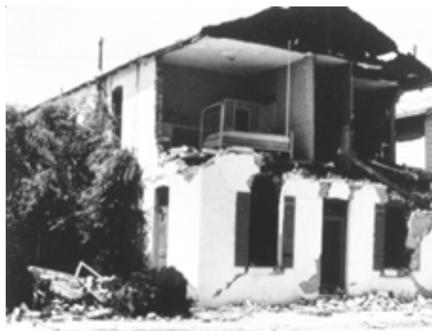
Figure 25 - The plaster-covered brick walls of this building collapsed during a recent earthquake.
