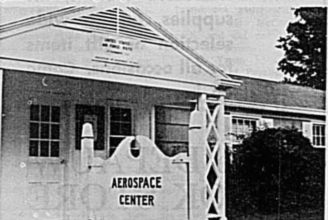
The Center as it looks today after an approximate $10 thousand remodeling job, provided by DePauw and the insurance company.
