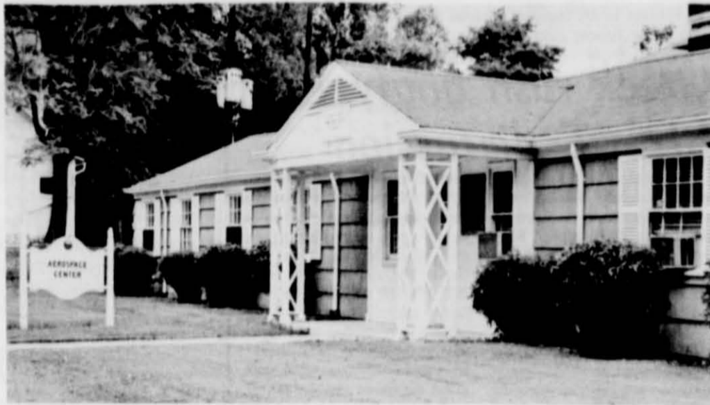
Will this building still be in use next year? —Photo by Emmerich
