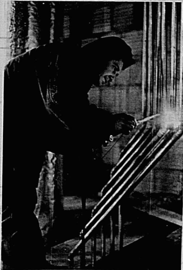
Steve Evan, a plumber from Indianapolis, is welding copper tubing to convey hot and cold refrigerants at a pressure of 150 lbs. per sq. inch. "People don't realize that their lives are in our hands," he said.
