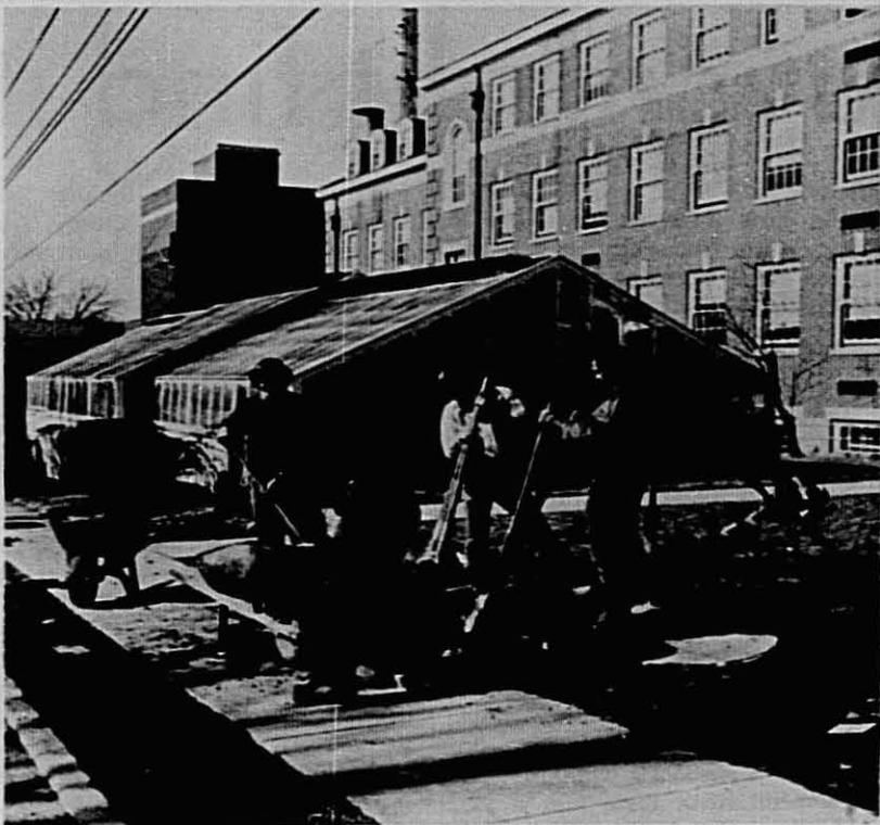
Workmen are laying the foundations and trenches for the new mercury vapor lights to be placed across campus. Installation is delayed until the fixtures and standards arrive.
