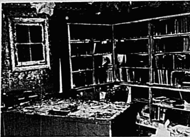
Charred books, desk, and files are all that remain in this office as an aftermath of Friday morning's ROTC fire.
