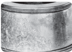
Inner race damage from misalignment. (fig. 5)
