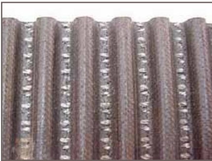
Figure 7 - Excessive land area wear
