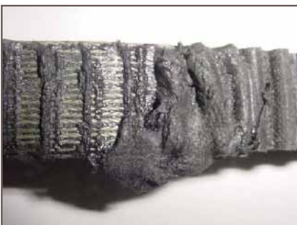
Figure 18 - Melting from high temperature operation, polyurethane
