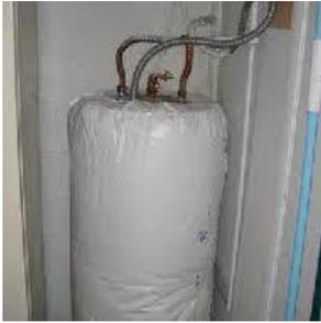
Unless your water heater's tank has a high R-value of insulation (at least R-24), adding insulation to it can reduce standby heat losses by 25 – 45%. This will save you about 4 – 9% in water heating costs.
