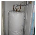
Unless your water heater's tank has a high R-value of insulation (at least R-24), adding insulation to it can reduce standby heat losses by 25 – 45%. This will save you about 4 – 9% in water heating costs.
