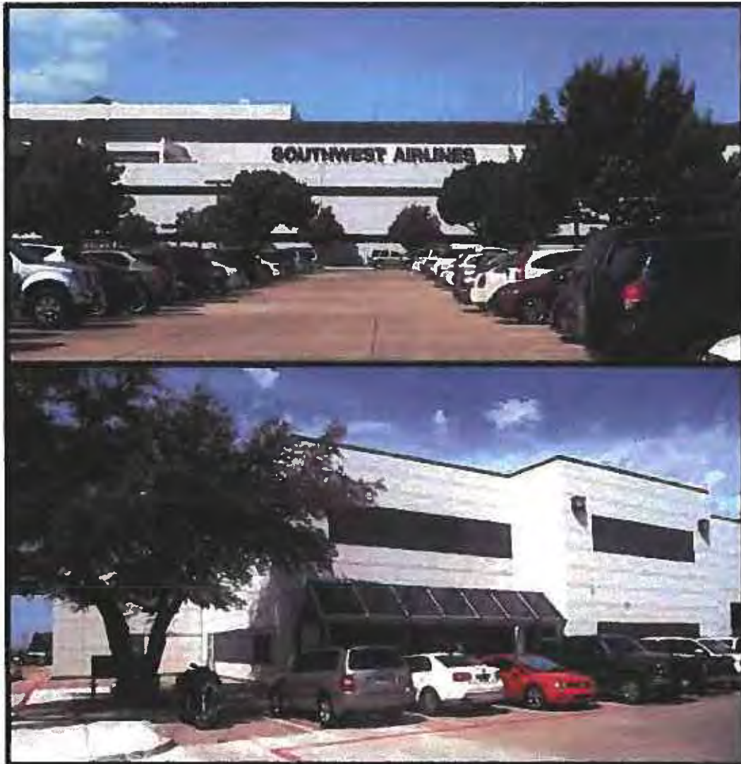
Source: Photographs taken by Ricondo & Associates, Inc., July 2012. Prepared by: Ricondo & Associates, Inc., April 2013
