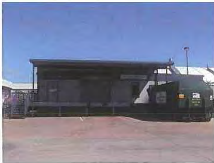
Source: Photographs taken by Ricondo & Associates, Inc., July 2012 Prepared by Ricondo & Associates, Inc., April 2013.
