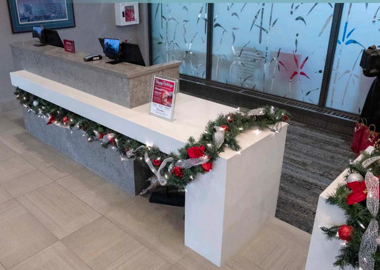
Precision fabrication was key—each desk includes mitered edge lamination for a seamless finish, and a carefully designed ledge running at varying heights. The result? A perfect blend of style and function, enhancing the welcoming experience for guests while showcasing the beauty and versatility of quartz stone.
