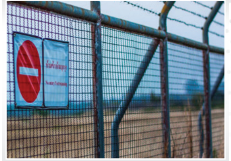
PERIMETER INTRUSION DETECTION (PID)
