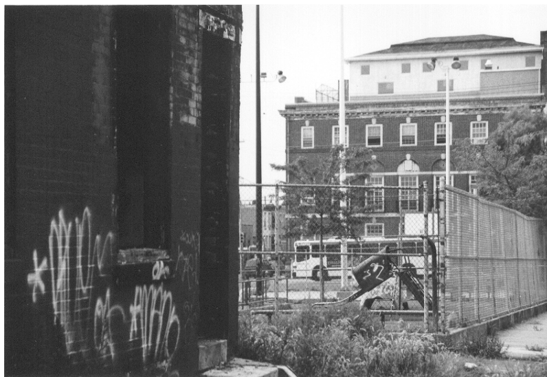
Photo 8: Open vacant house less than twenty feet from McGuire Playground at Mutter Street & Lehigh Avenue. Across the street is the Light-house Community Center. Photo taken September 2001.
