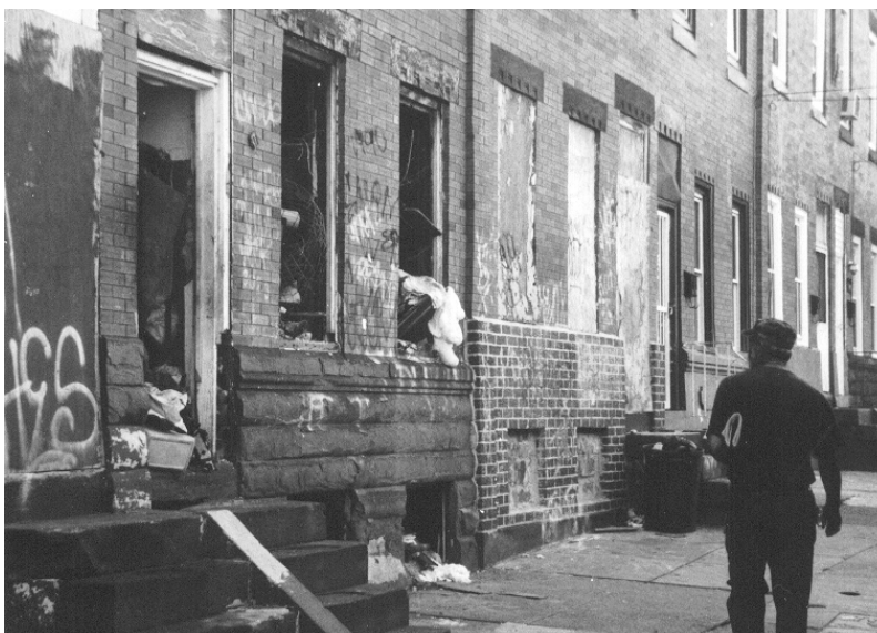
Photo 3: One of a string of four vacant houses at the center of this residential block in West Kensington. Photo taken September 2001.
