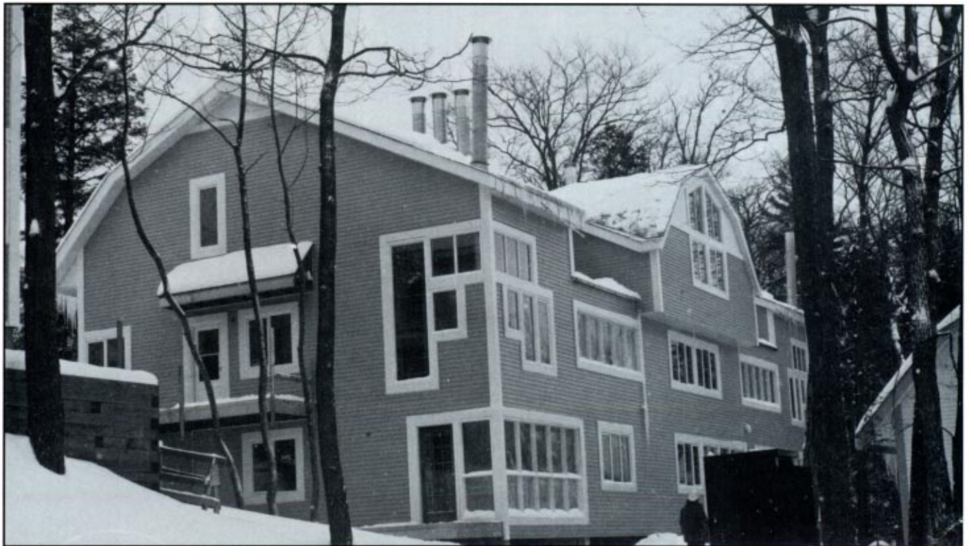
AFTER The building after application of exterior grade sheathing and finished with metal siding. The Bailey/Mantane steel framing systems are compatible with most exterior cladding materials such as brick, stucco, siding etc.
