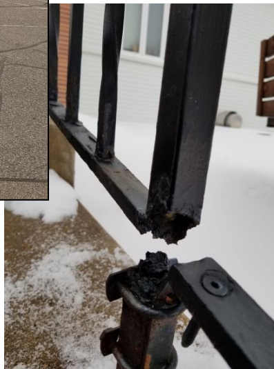
Picture above: parking lot showing it's wear. Pictured right: Stair railing in the front of the church rusted through.
