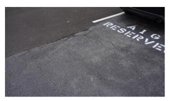
As a rule of thumb, asphalt should be overlaid when approximately 5% of the surface area is cracked or otherwise deteriorated. The normal service life of asphalt pavement is typically 18 to 20 years.
