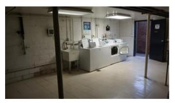
The condition of these light fixtures ranges from good to poor, as some fixtures appear to be newer or have been retrofitted with LED luminaries while others are in poor condition with inoperative luminaries and stained diffusers noted.
