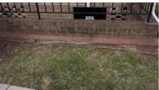
The brick retaining walls are primarily located at the below-grade access ways to the laundry rooms and storage rooms at either end of each of 12 buildings and at one end of three buildings. The condition of these walls varies from good to poor, with the primary deficiencies being loose and missing mortar, loose and missing brickwork, loose and deteriorating brickwork at metal railing bases, through-wall cracking, and deterioration of surface parging.
