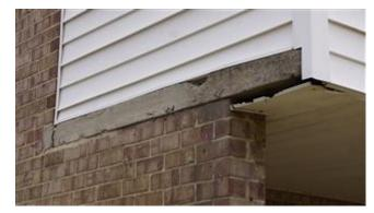
Concrete balconies are prone to deterioration due to their exposure to the elements. This deterioration begins within the concrete and slowly progresses to the surface. By the time it becomes visible, the damage has been done, and expensive remedial action is typically required.
