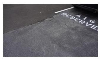
As a rule of thumb, asphalt should be overlaid when approximately 5% of the surface area is cracked or otherwise deteriorated. The normal service life of asphalt pavement is typically 18 to 20 years.
