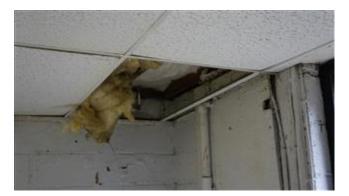
It is important that the integrity of these ceilings tile be maintained as it helps to insulate the above spaces to protect piping installed above the tile. Any gaps or missing tile will allow cold air to penetrate the space above the tile, increasing heat loss from the conditioned space increasing the chances of freezing the piping above the tile. We recommend that the tile be inspected in the fall and after any work is completed in the space above the tile.
