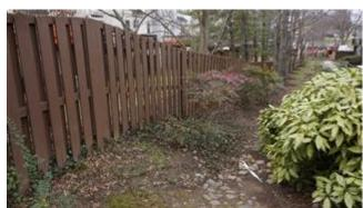
The wood board-on-board fencing is located along portions of the southwest property line, around the play area, at the trash enclosures at each of the 15 buildings, and at privacy fences at certain individual townhouse units. The condition of these various fences varies from good to poor, with rotten components, loose fence posts, and out of plumb sections of fencing noted
