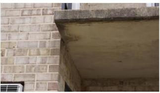
We noted no major defects which appear to be significant, although cracking in the concrete decks near support structures, cracks in supporting brick masonry, and spalling of brick at balcony bearing locations is noted. These defects should be closely monitored to determine if any of these conditions worsen over time.
