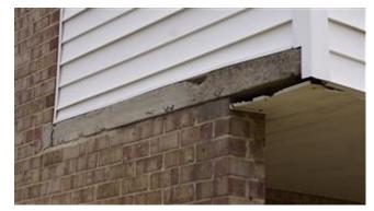
Concrete balconies are prone to deterioration due to their exposure to the elements. This deterioration begins within the concrete and slowly progresses to the surface. By the time it becomes visible, the damage has been done, and an expensive and extensive remedial action is typically required.
