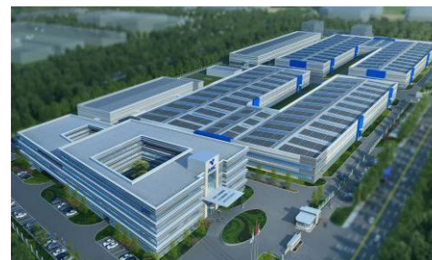
Jiangxi Shangrao factory 9GWh business car power&ESS battery production base Geely Farizon business car, Changan business car, Xiongtao, Shuangdeng Group
