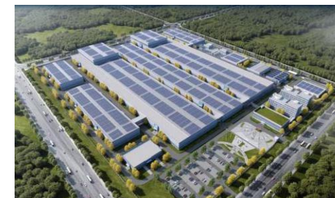
Jiangxi Yingtan factory 6GWh business car power&ESS battery production base Wuling business car, Ruilan battery change Star Energy Technology
