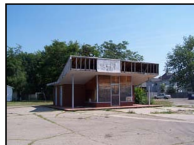
This abandoned gas station is a prime candidate for brownfield investigation due to the possibility of contamination.
