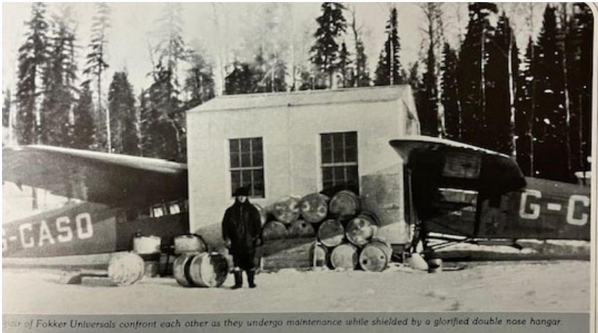
pair of Fokker Universals confront each other as they undergo maintenance while shielded by a glorified double nose hangar
