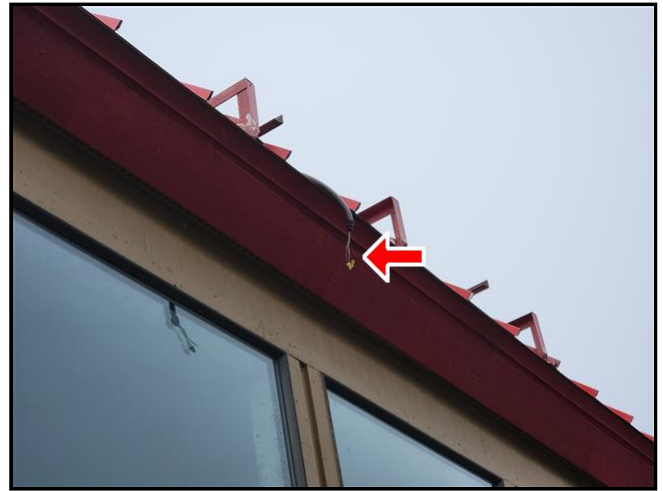
6.3 Item 6(Picture) East side of building.
