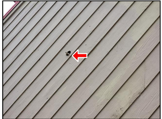
6.3 Item 8(Picture) North side of building.
