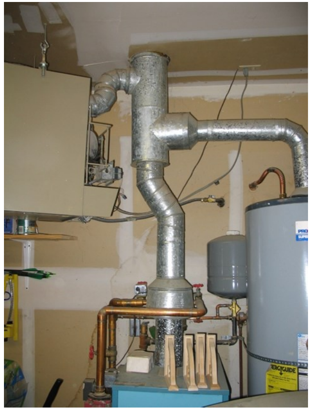
Appliance connectors entering at different levels.
