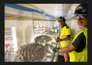
Five auxiliary cold boxes at Level 3 of the Tokamak Building have been connected to cryolines and testing is underway. The 28-tonne components act like dispatchers, receiving the different fluids from the cryogenic termination cold box located inside the cryoplant and redistributing them throughout the ITER machine.
