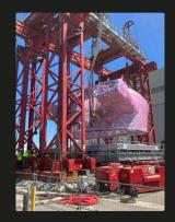
Another sector rotated outdoors. After vacuum vessel sector #4 in June, sector #1 has been rotated under the huge gantry crane that has been installed on the platform near the former Cryostat Workshop
