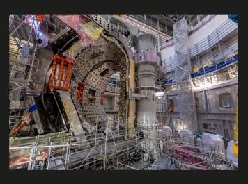
Sector modules #6 and #7 were installed in June and April, respectively. Another sector module should be inserted in December.
