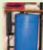
cold water tank installed in the loft
