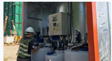
充足淨空高度 Sufficient Working Headroom
