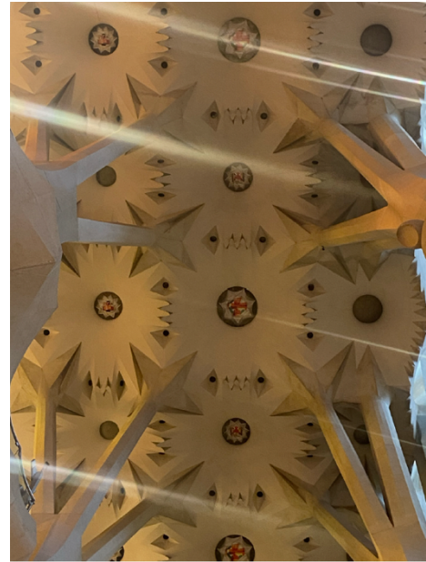
Figure 5 - The ceiling of the church where we can see the intersection of two doubly ruled surfaces
