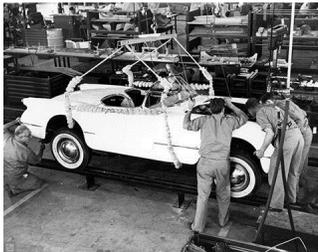
!Its radical fiber-glass body was the only really new component on the 1953 Corvette. Everything else was directly off the Chevrolet parts shelf. Because of this, the first Corvette was essentially a regular 1952 Chevrolet
