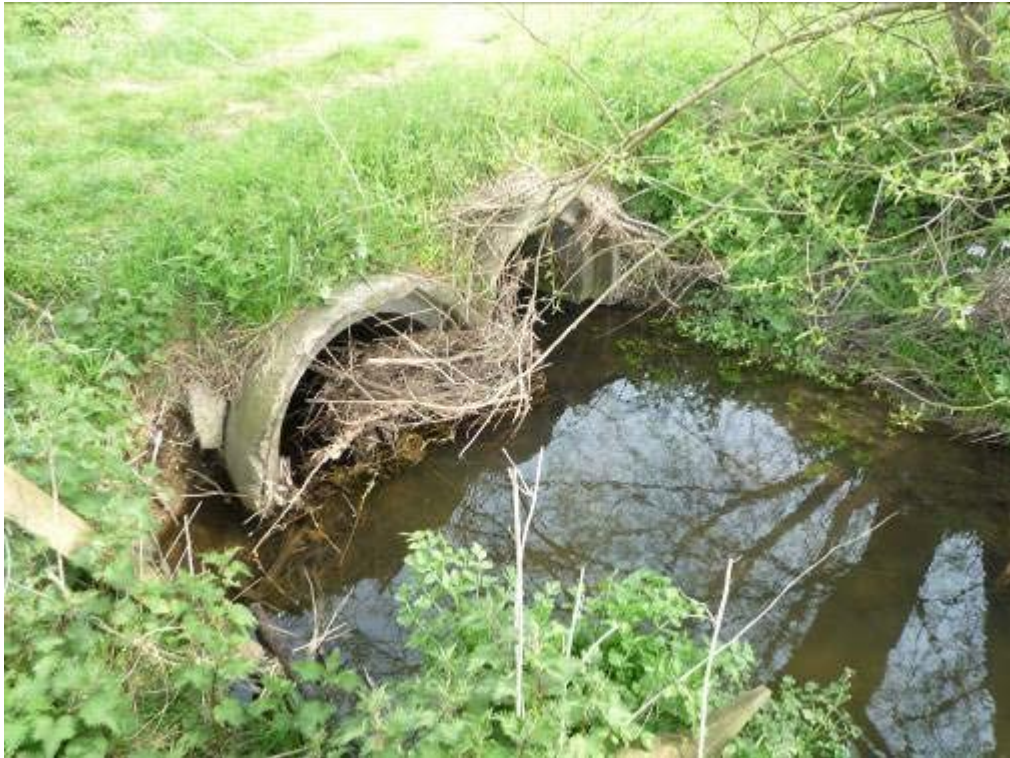
Blockage on the upstream end of the stream culvert. An open channel and clear span bridge may encourage fish to run the stream.
